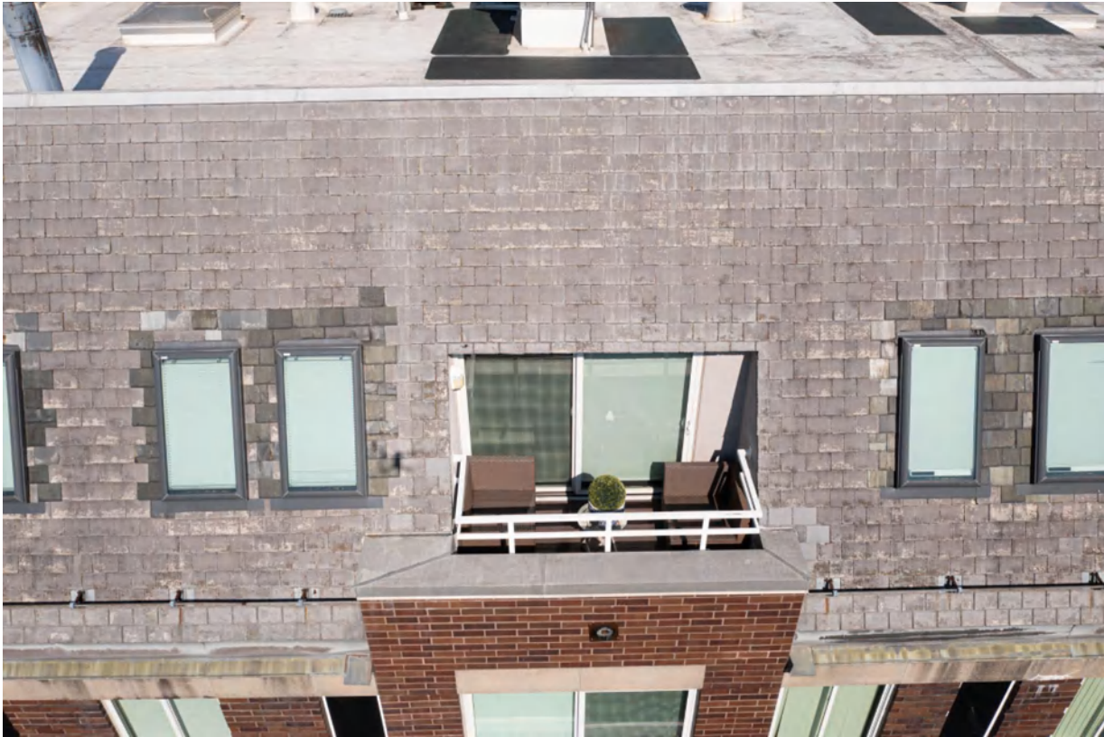
Photo 10: replaced shingles (with what appeared to be natural slate shingles) at localized locations around skylights
