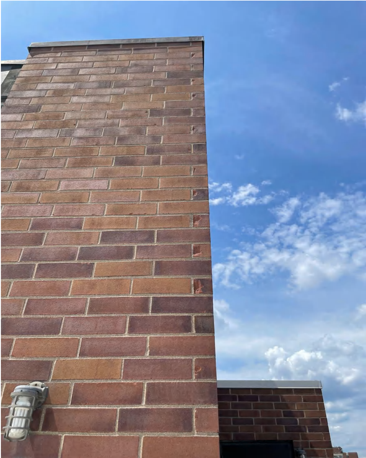
Photo 4: cracked, chipped bricks at corner of the west roof penthouse screen wall
