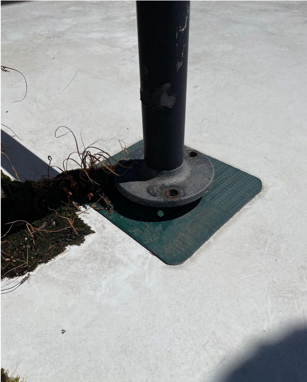
Photo 8: balcony railing post bases loosely set (without fasteners) and missing small 5/4" pressure treated roof sleeper block with welded walk pad
