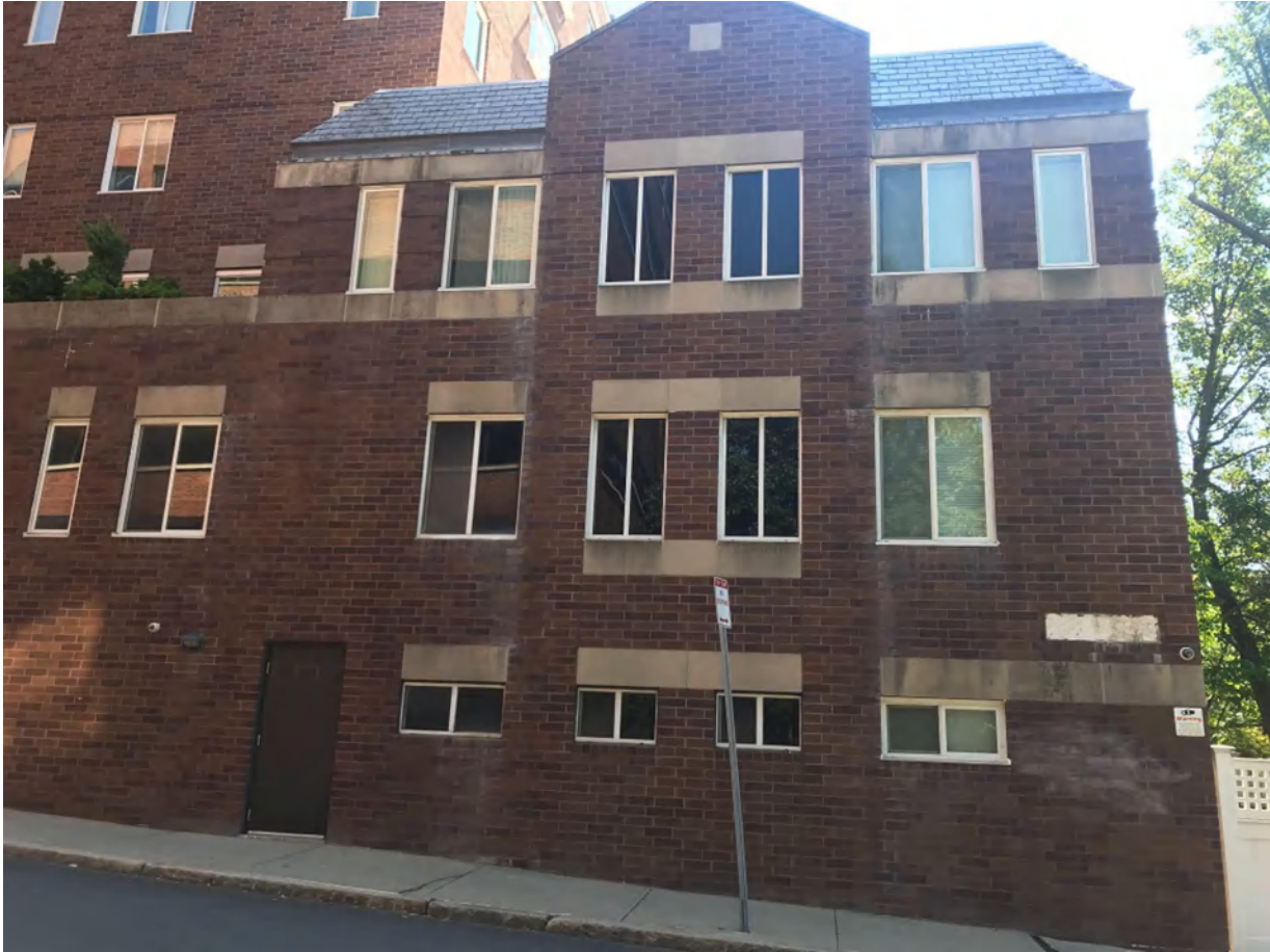
Photo 21: brick and cast stone staining at areas directly below mansard roof edge/dormer rising wall interface areas and below roof edges without gutters
