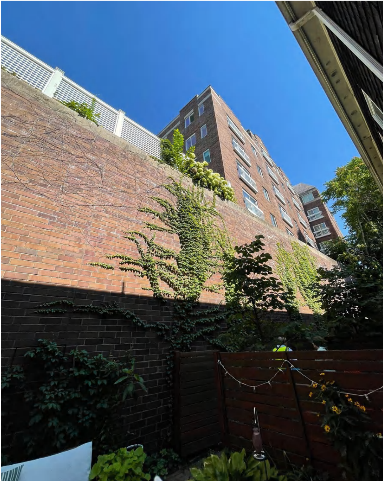
Photo 15: ivy growth on wall at east elevation
