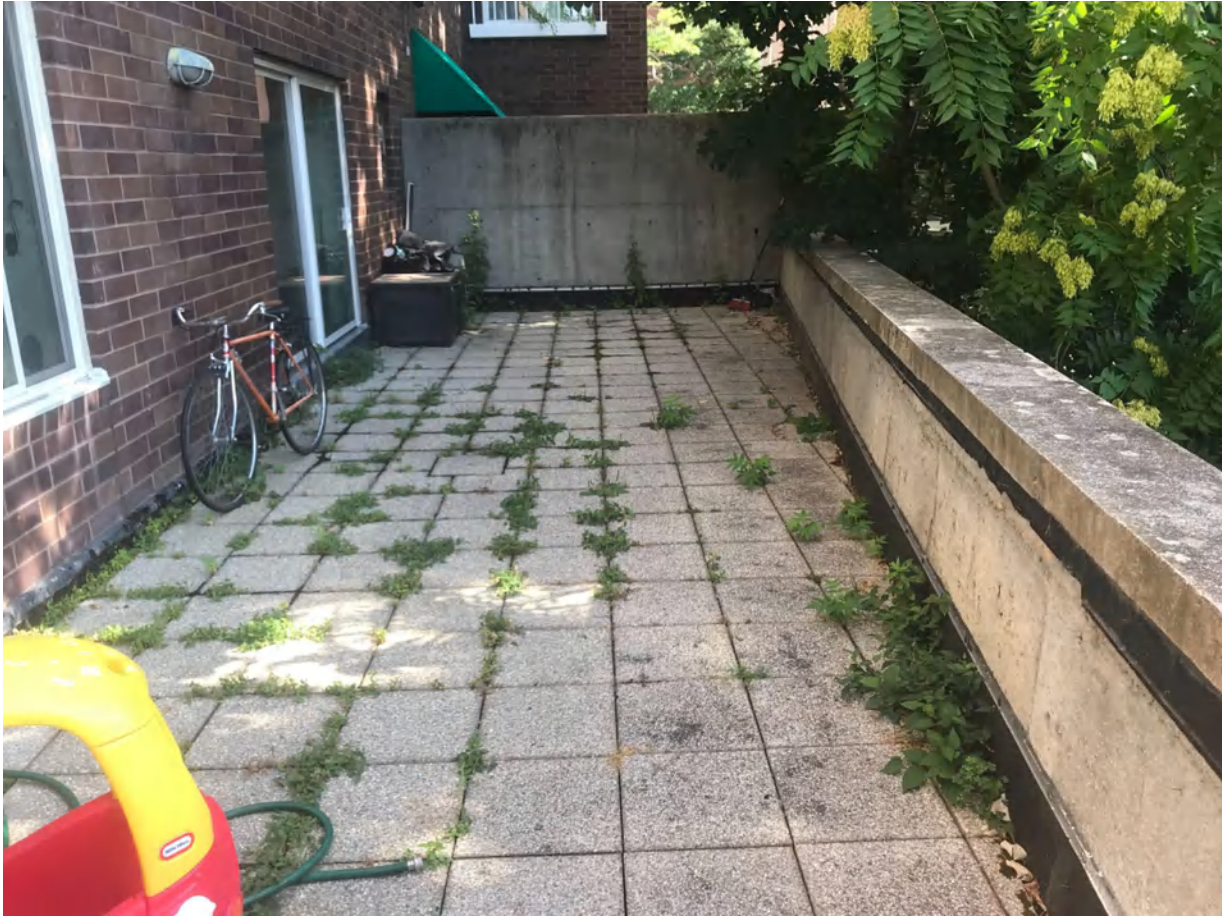
Photo 42: weed growth at the overburden surfaces and perimeter areas of Unit 106 terrace - original 1989 construction
