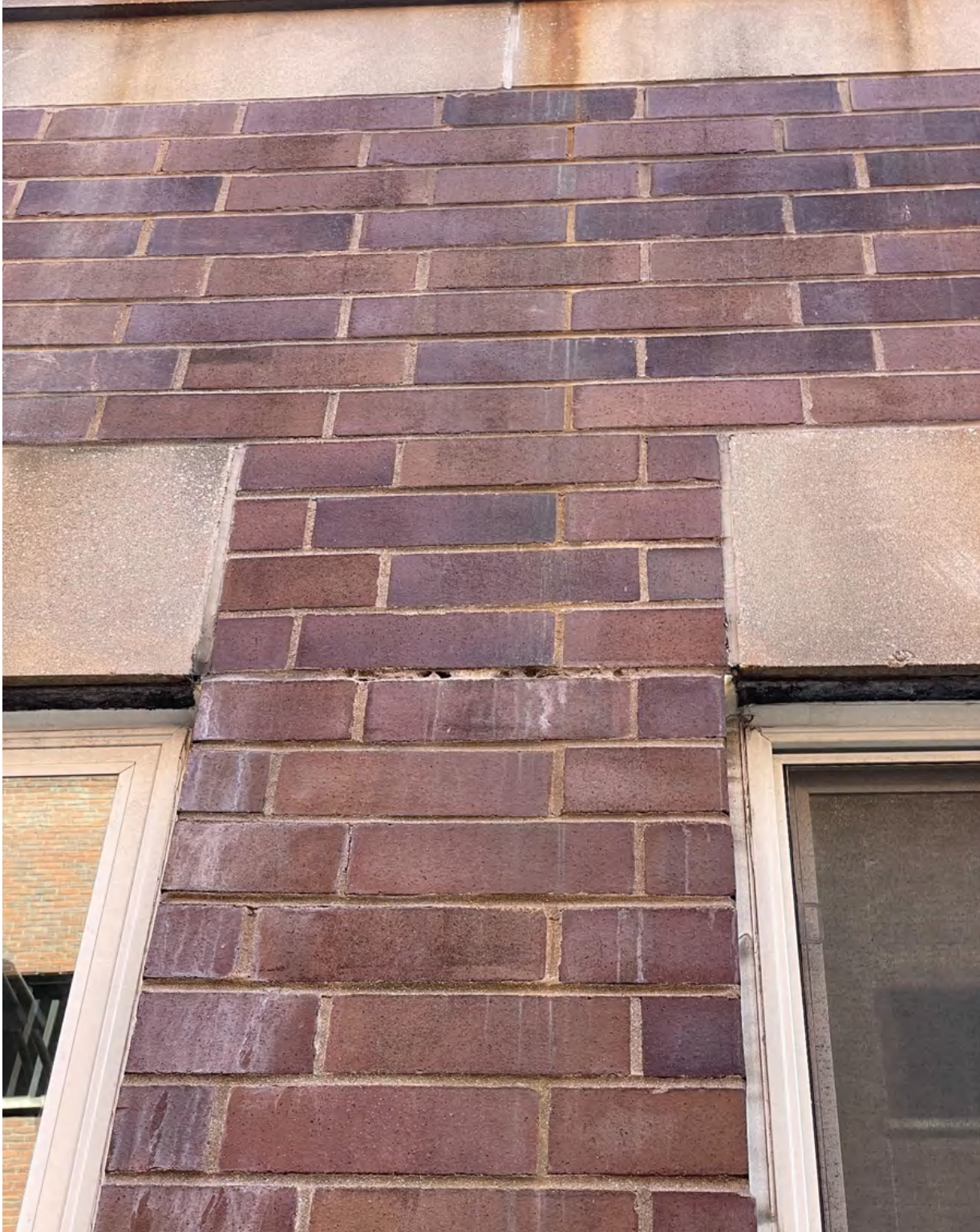
Photo 22: exposed areas of the galvanized steel relieving angles over the windows and failing joint sealant
