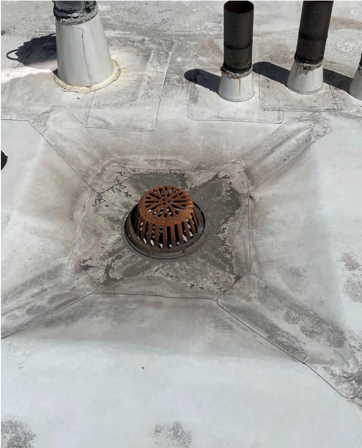
Photo 6: delaminated roof membrane at the roof drain sump and rusted roof drain components
