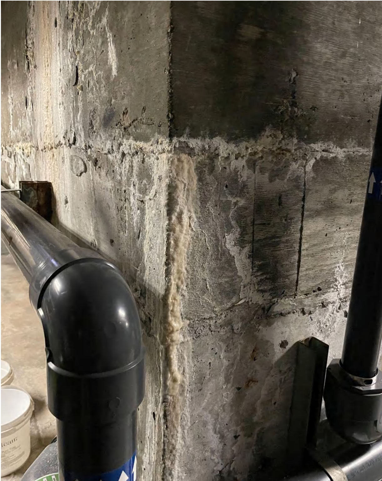
Photo 47: leak source appears to be from cold joint at the pool wall and lower slab
