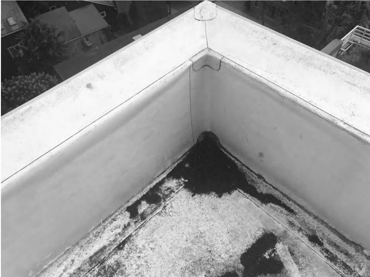
Photo 2: organic build-up on white reflective roof membrane surfaces in random locations
