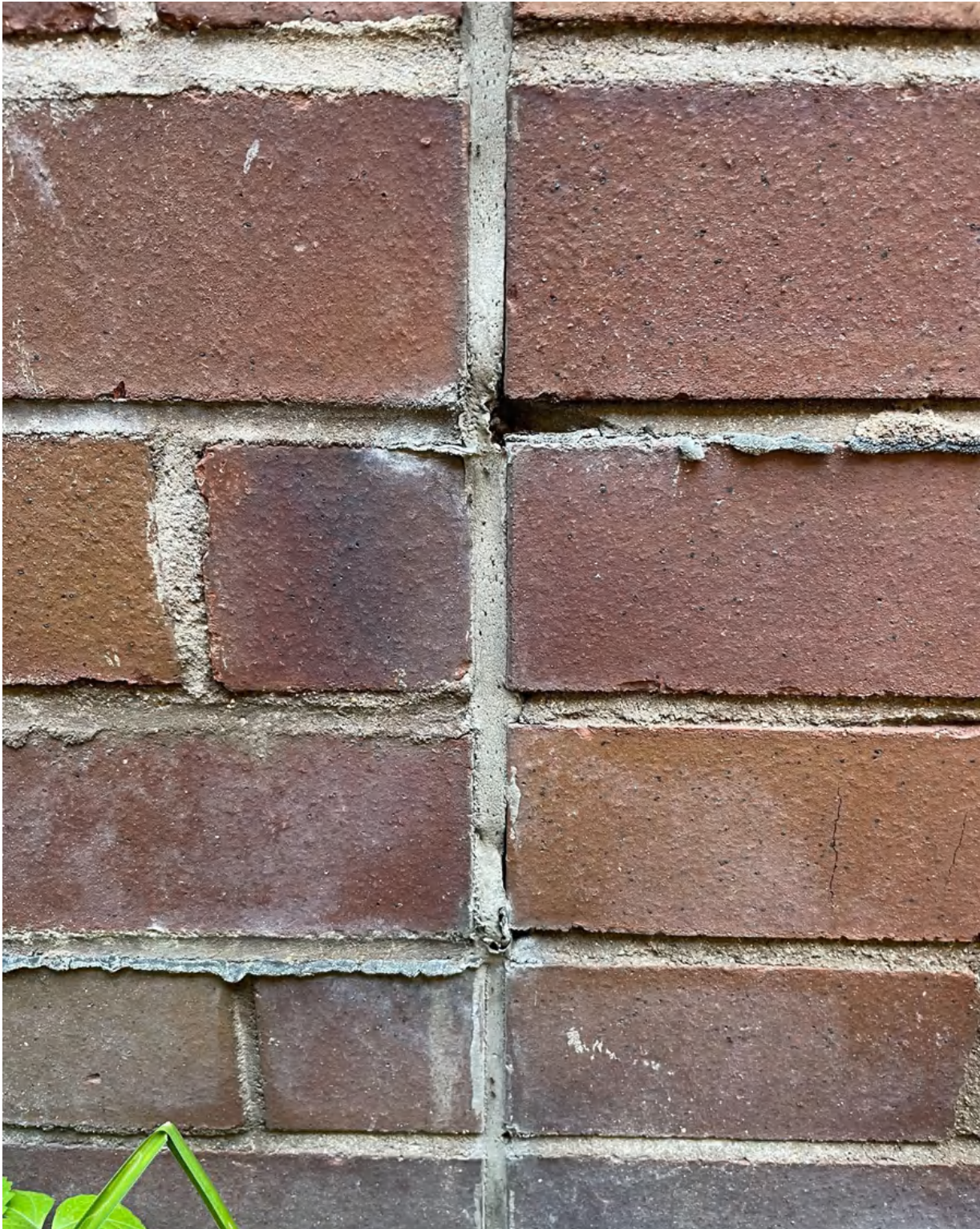
Photo 24: failing control joint at the east elevation wall that abuts the 551 Green Street
