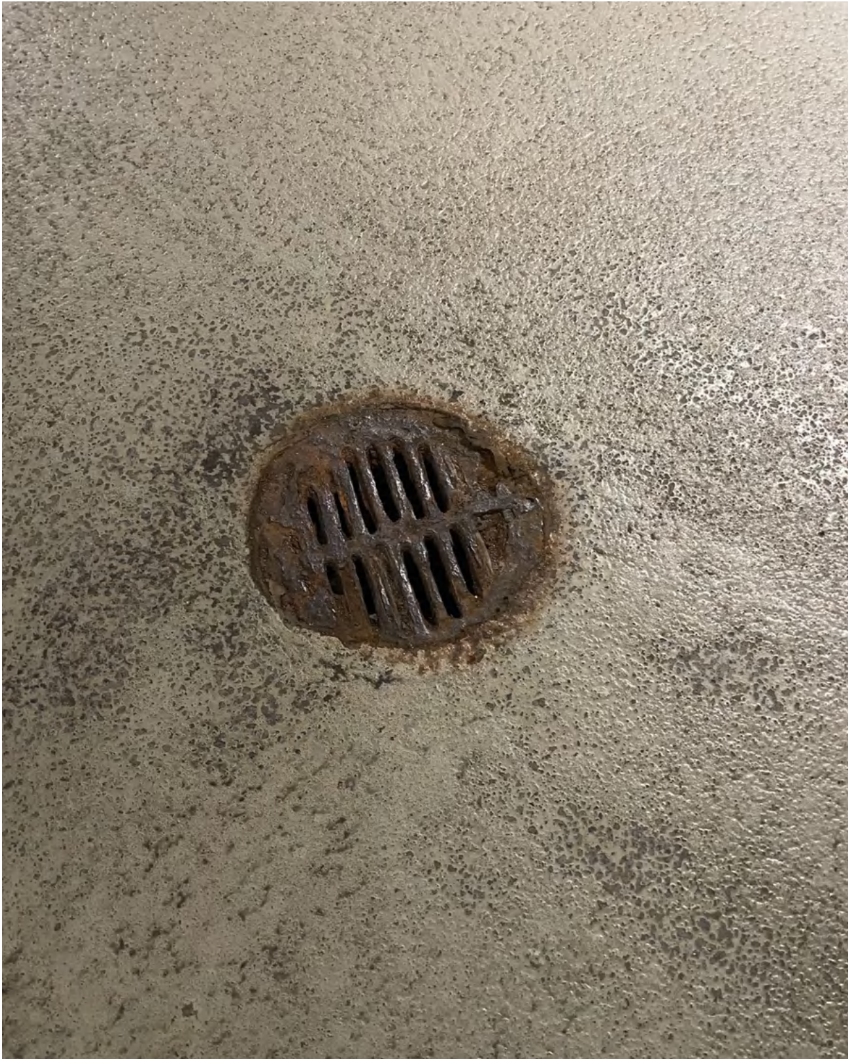
Photo 40: severely rusted/aged garage floor drain (appears to be the original to the 1989 garage)
