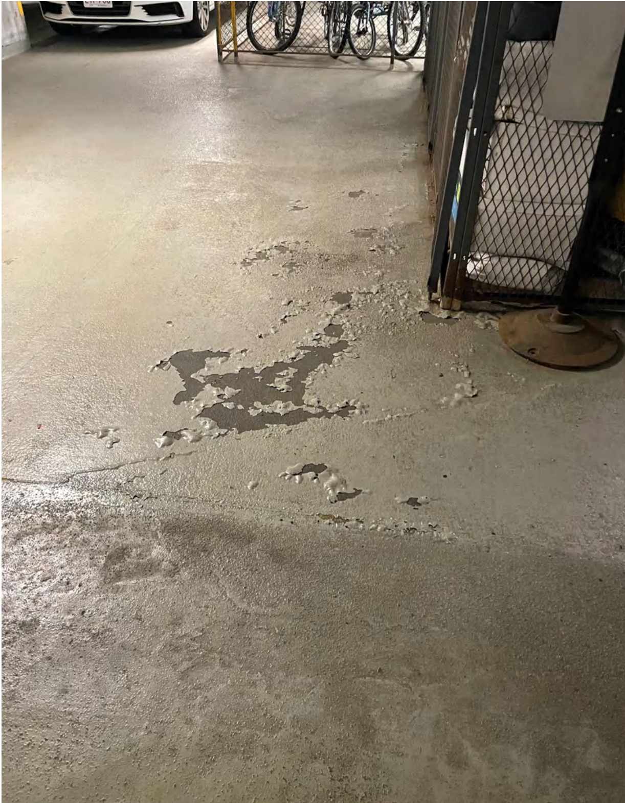
Photo 37: delaminated urethane traffic coating at the upper level garage
