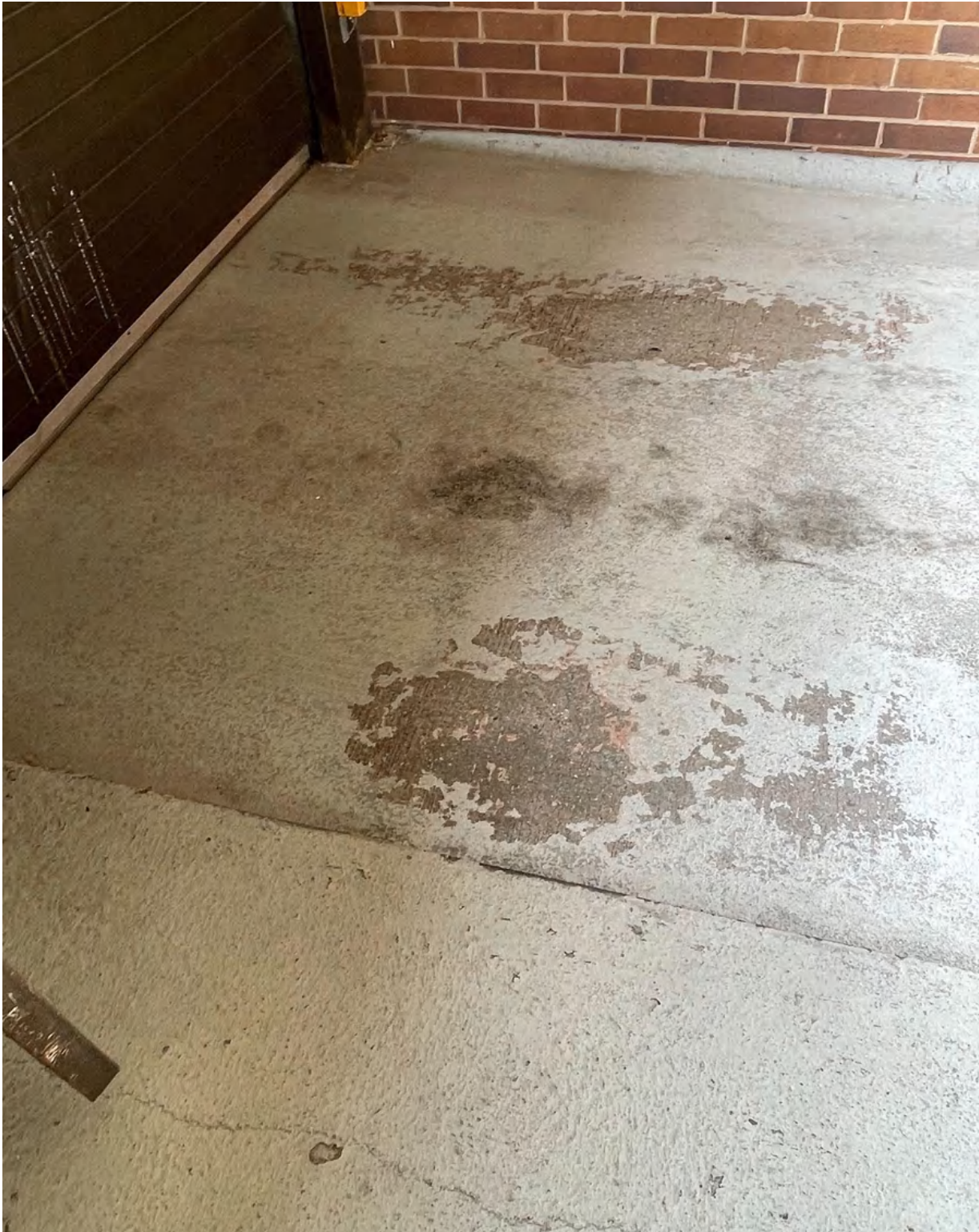
Photo 39: worn out/delaminated urethane traffic coating at the upper level garage driveway entrance
