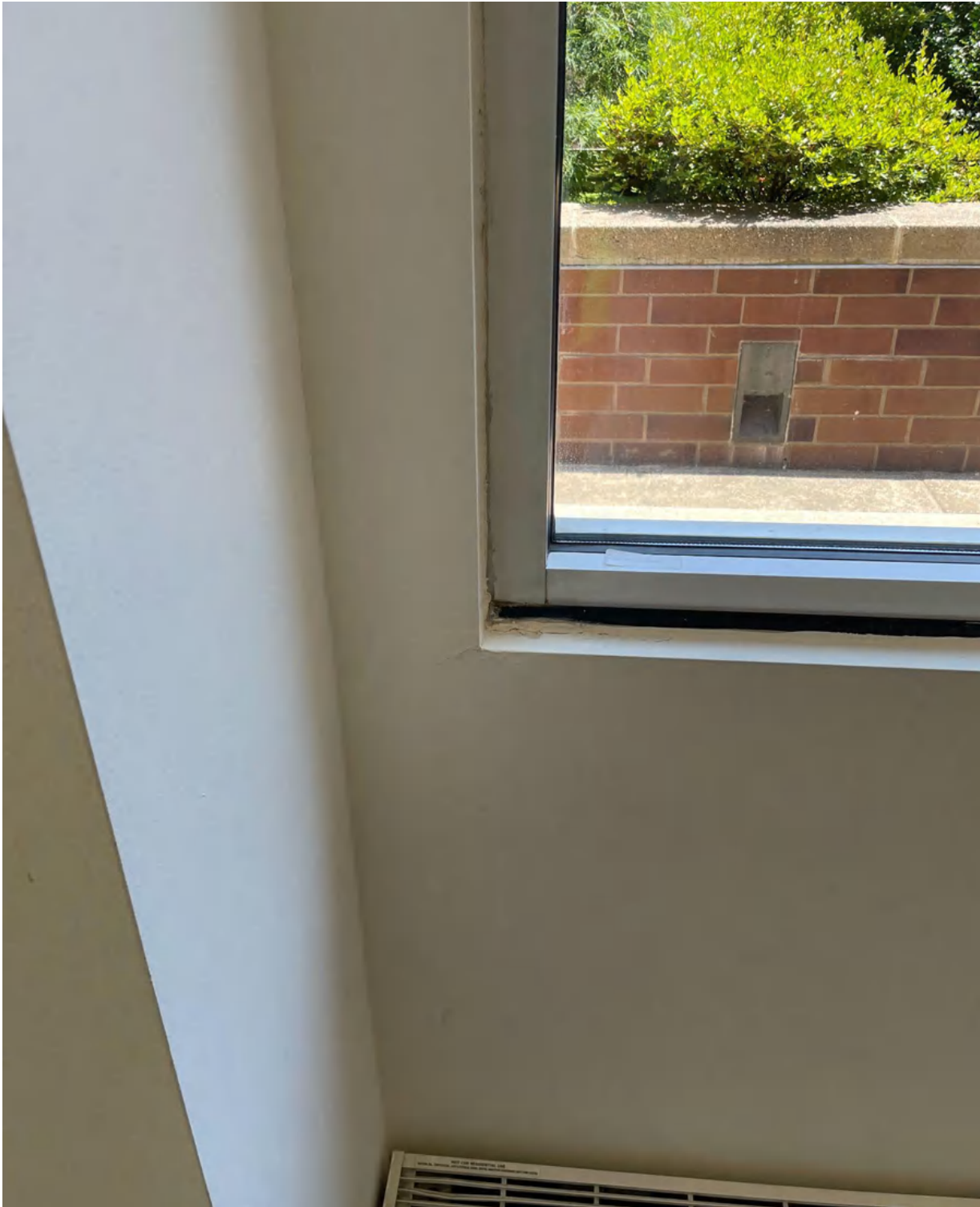
Photo 28: window sill at lobby hall area where facilities staff reported of water leaking history
