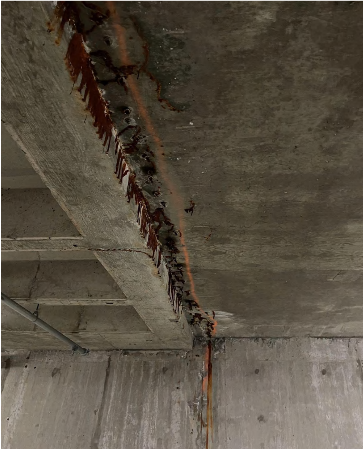
Photo 41: grout injection ports from remedial repairs in the past at ceiling of Upper Garage
