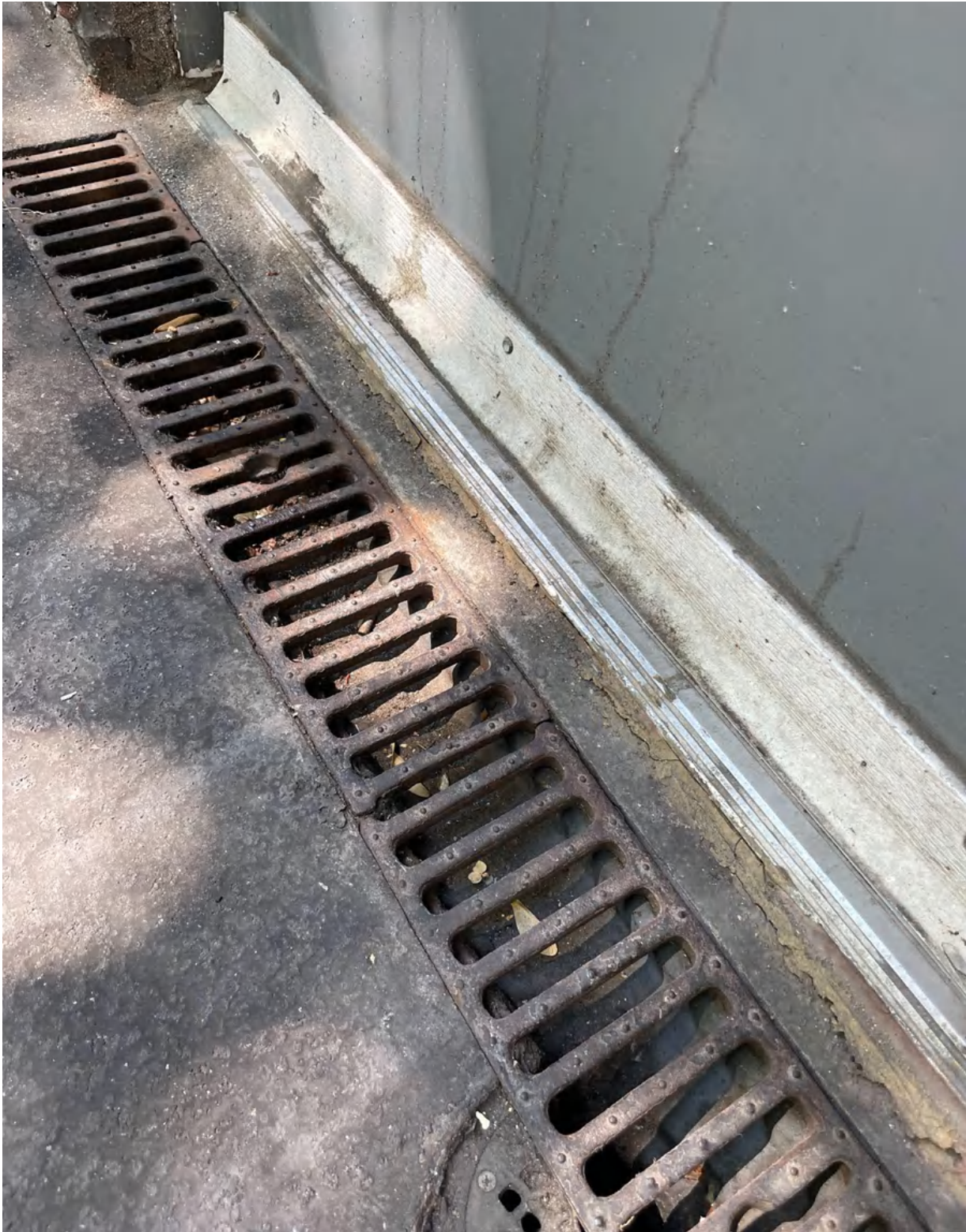
Photo 29: failing threshold sealant at loading dock doors & aged retrofit trench drain
