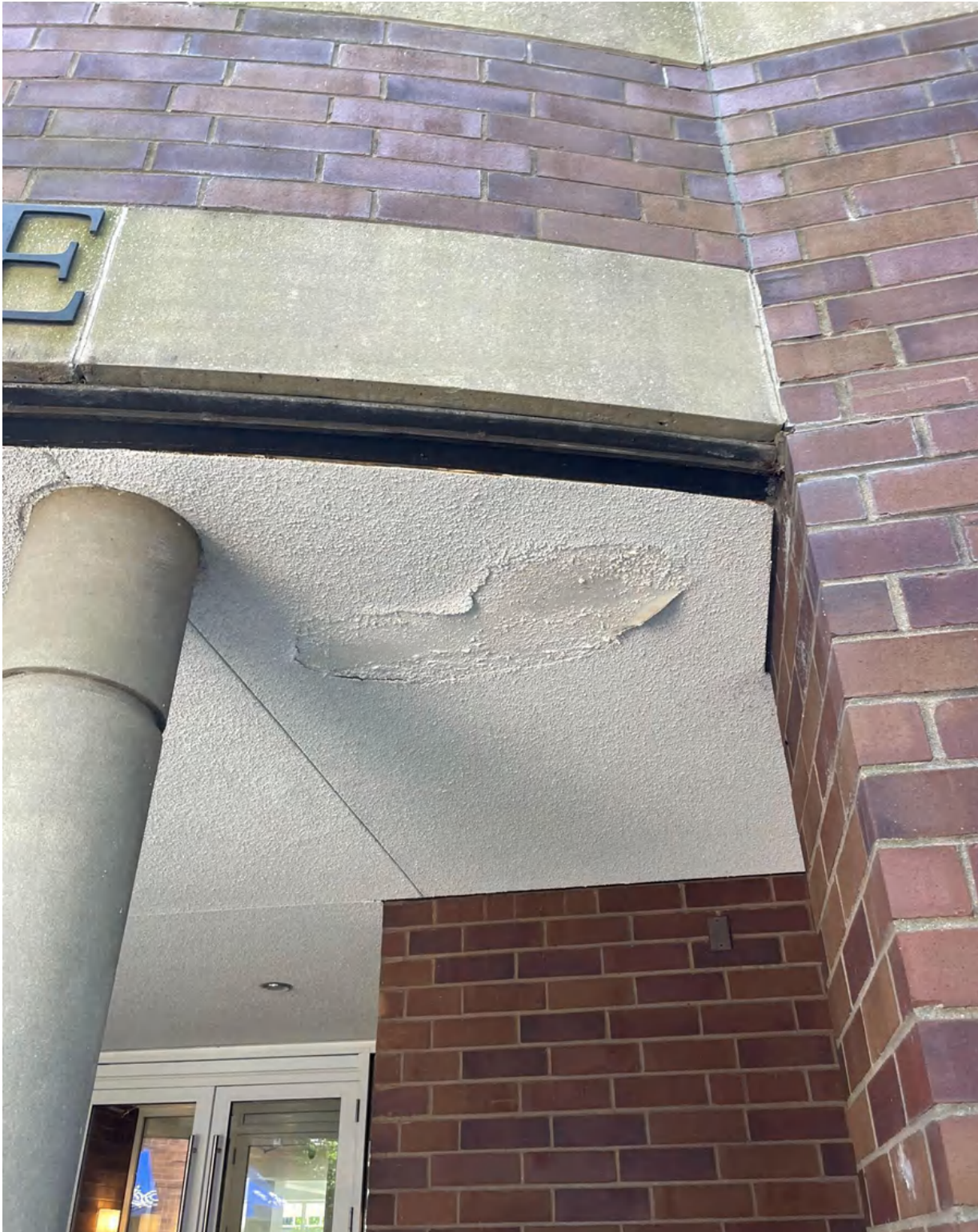
Photo 23: peeling stucco finish at the main entry portico soffit reported from previous balcony leaks (waterproofing/roof above now replaced)
