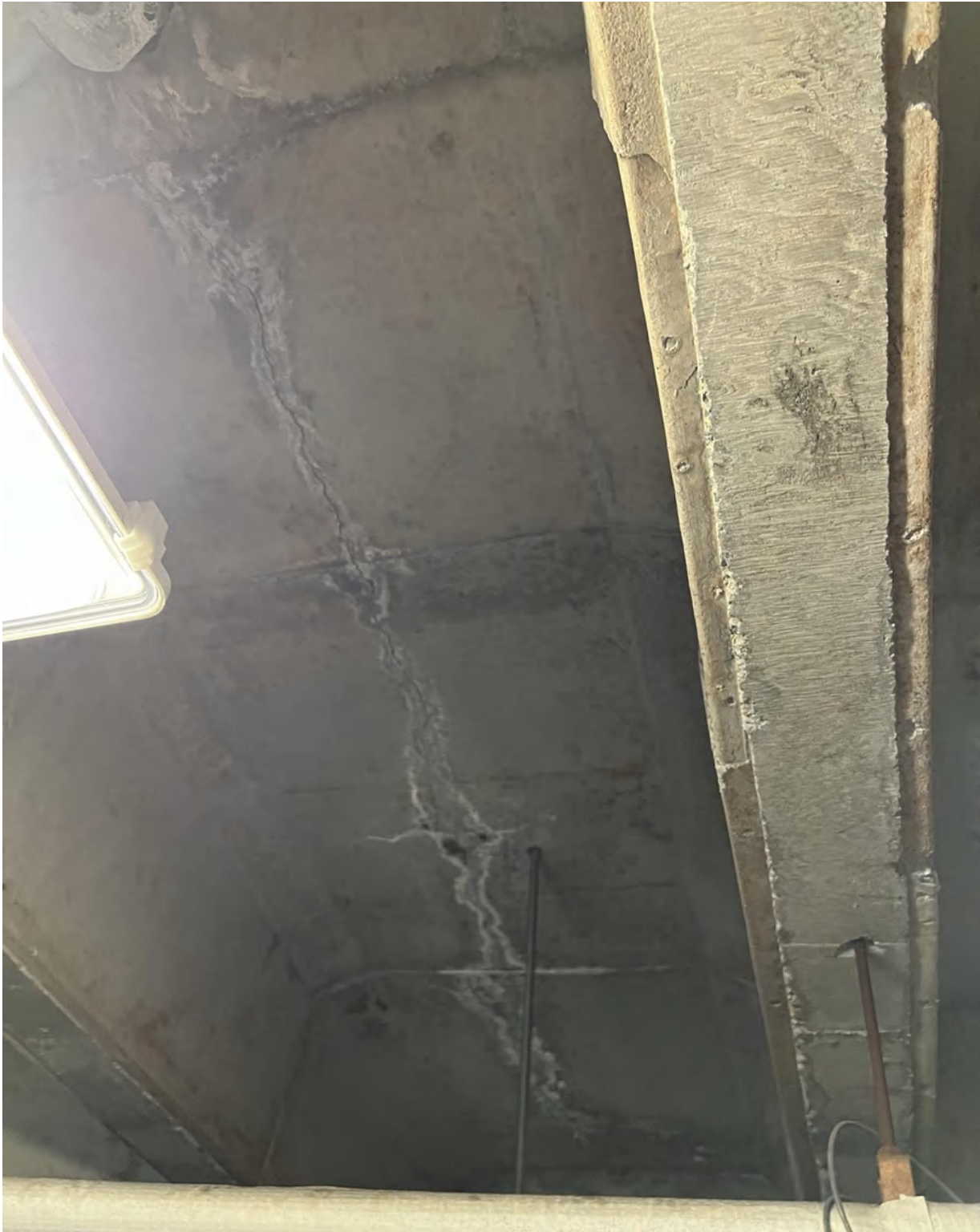
Photo 35: cracking at the concrete waffle slab ceiling with water leakage staining
