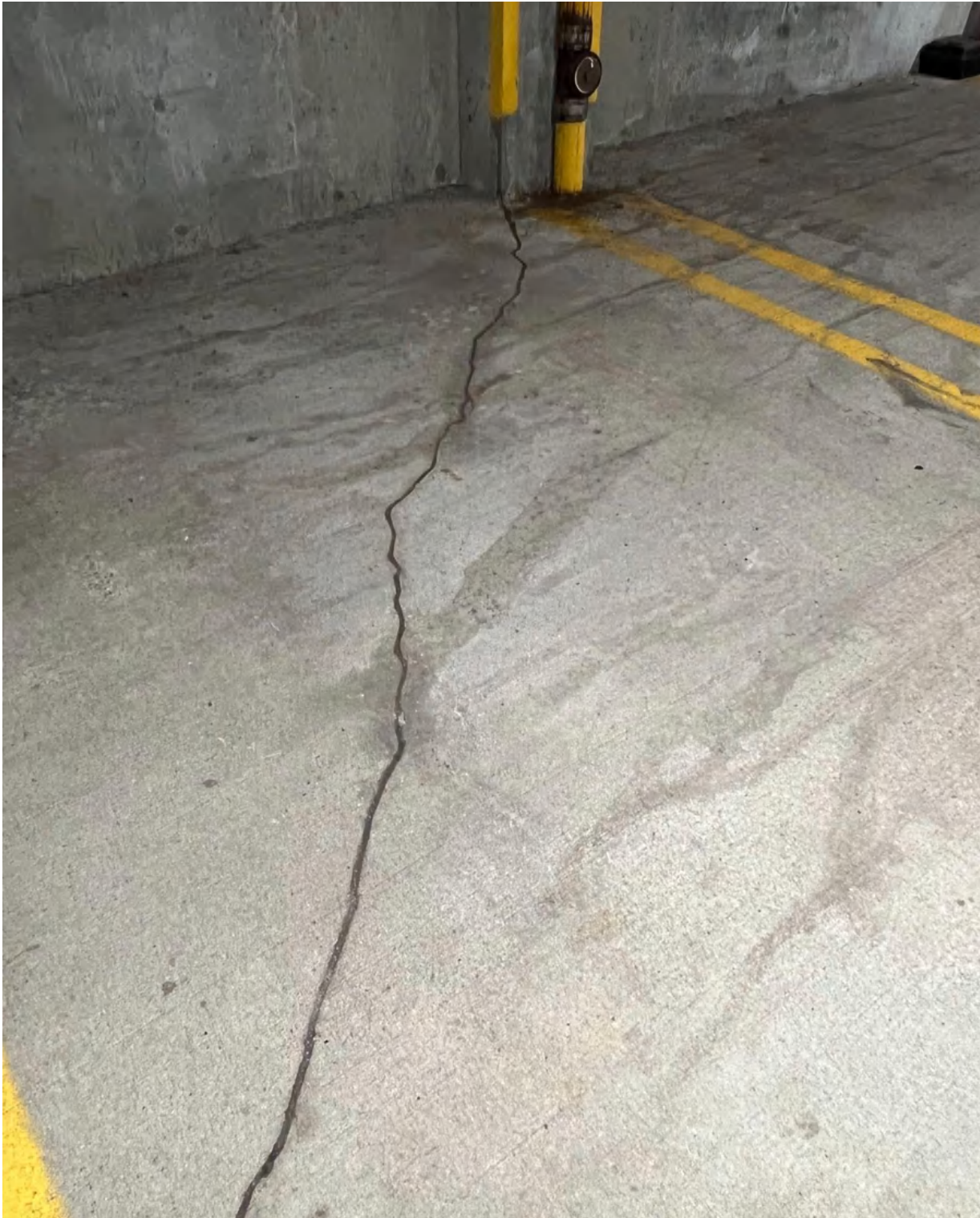
Photo 31: slab cracking with “rout & seal” sealant repair observed on floor slabs at parking stall
