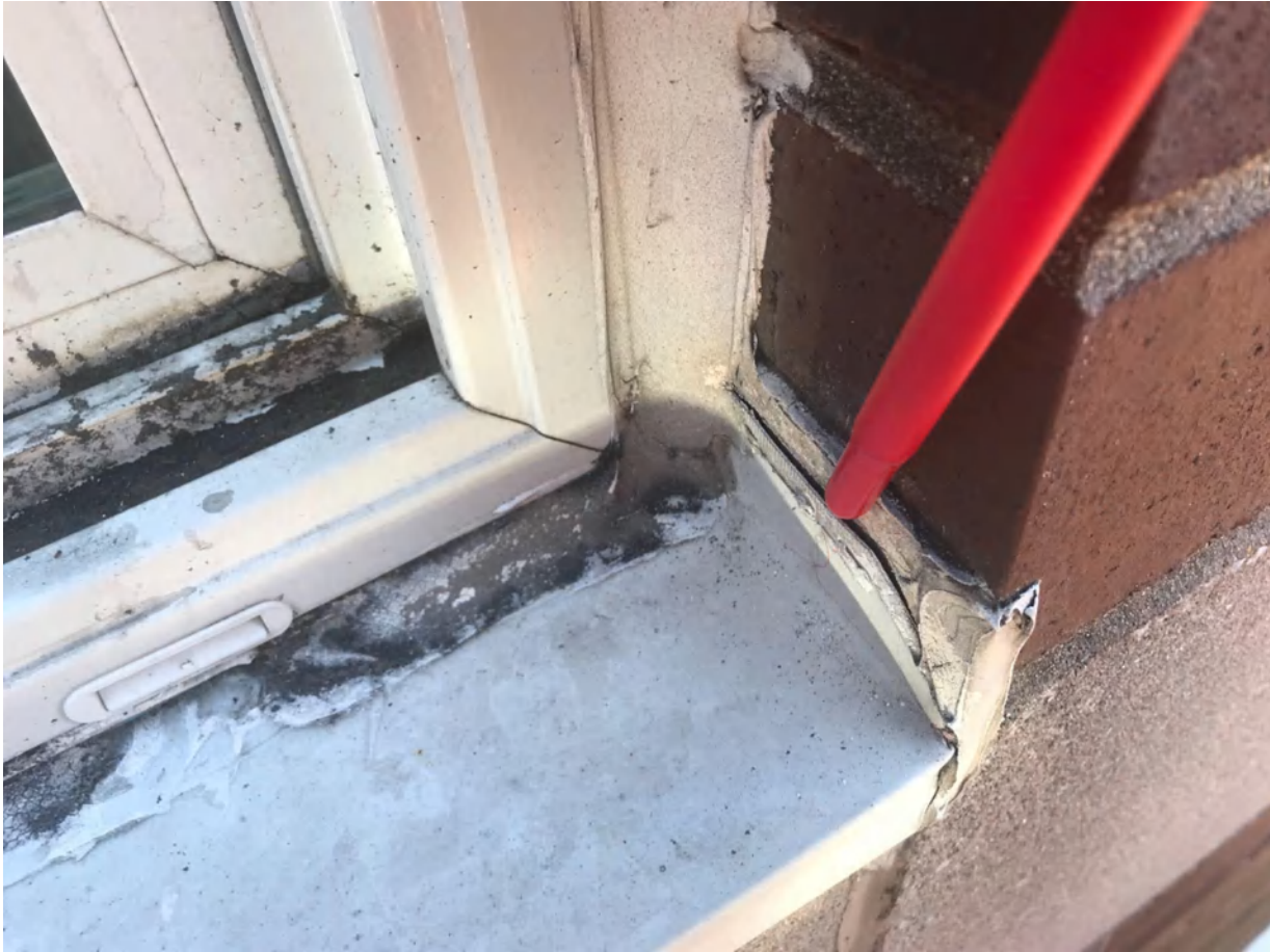
Photo 26: failed sealant joint at the windowsill aluminum pans at the turn-up to the brick jambs at 6th floor level - north elevation
