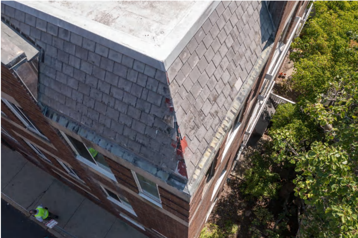
Photo 13: damaged/missing shingles at the southwest hip area of the steep sloped mansard style roof from reported tree impact
