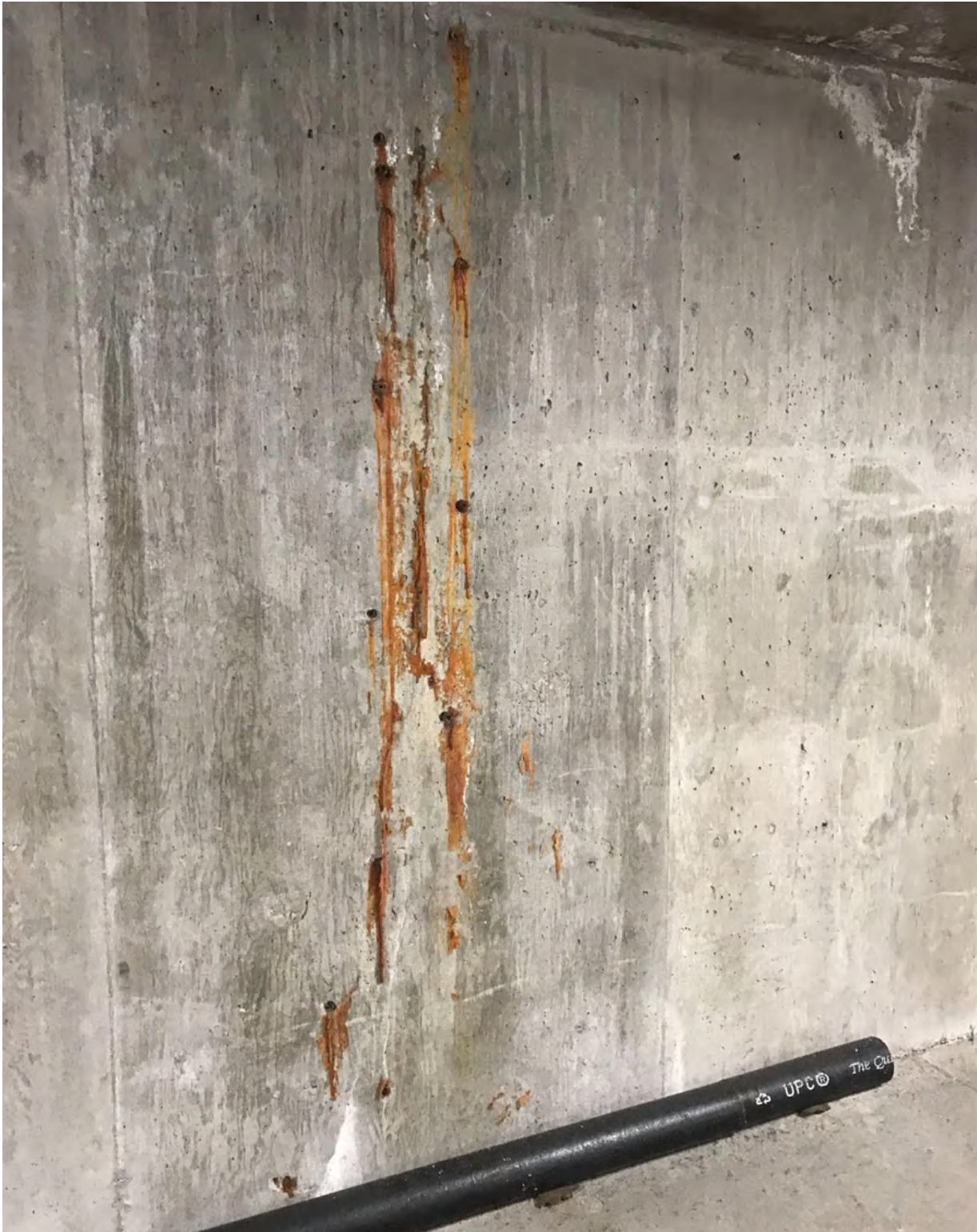
Photo 34: signs of previous negative side remedial waterproofing repairs at garage wall on the east end
