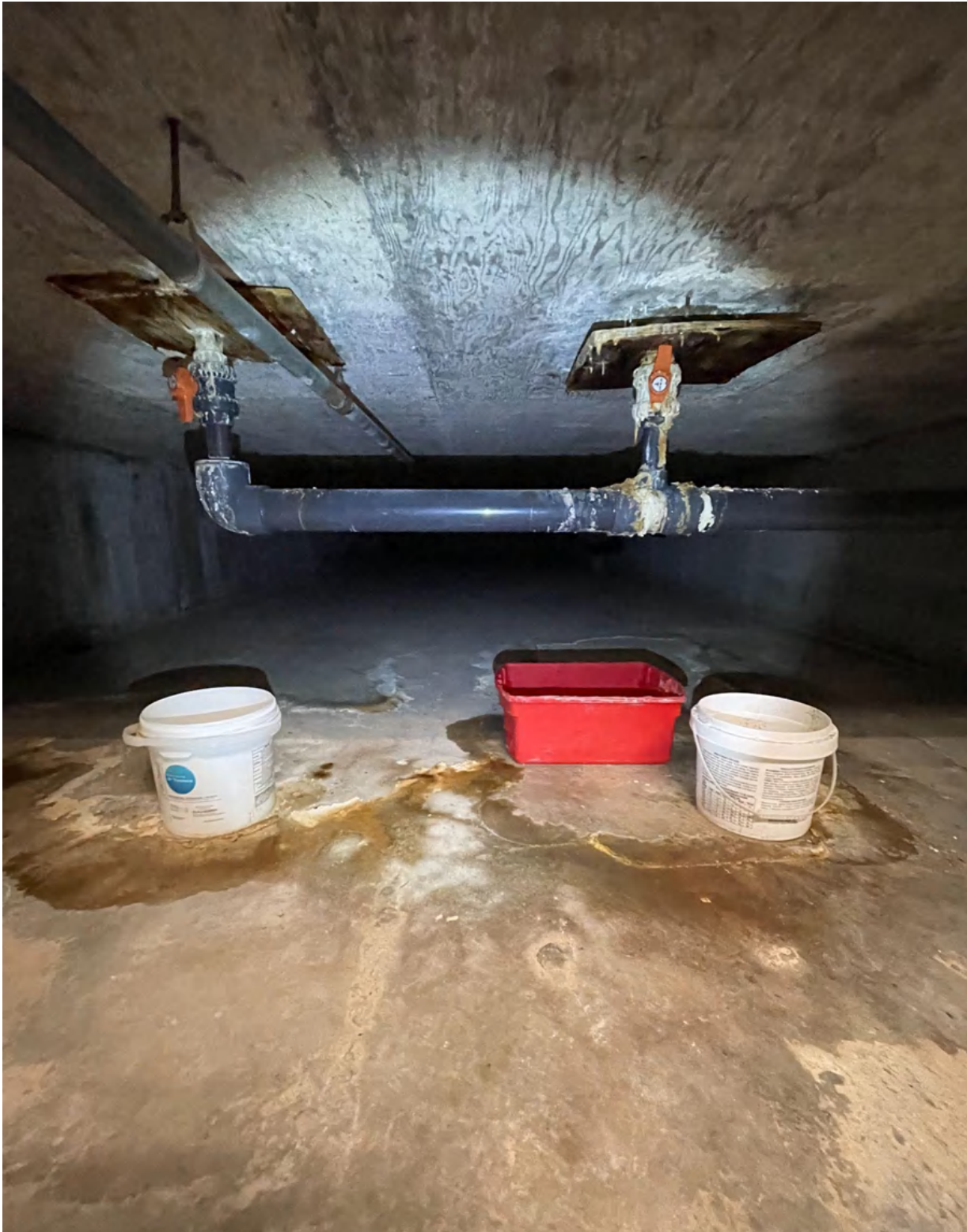
Photo 48: active leak at conduit penetration through bottom slab of the pool
