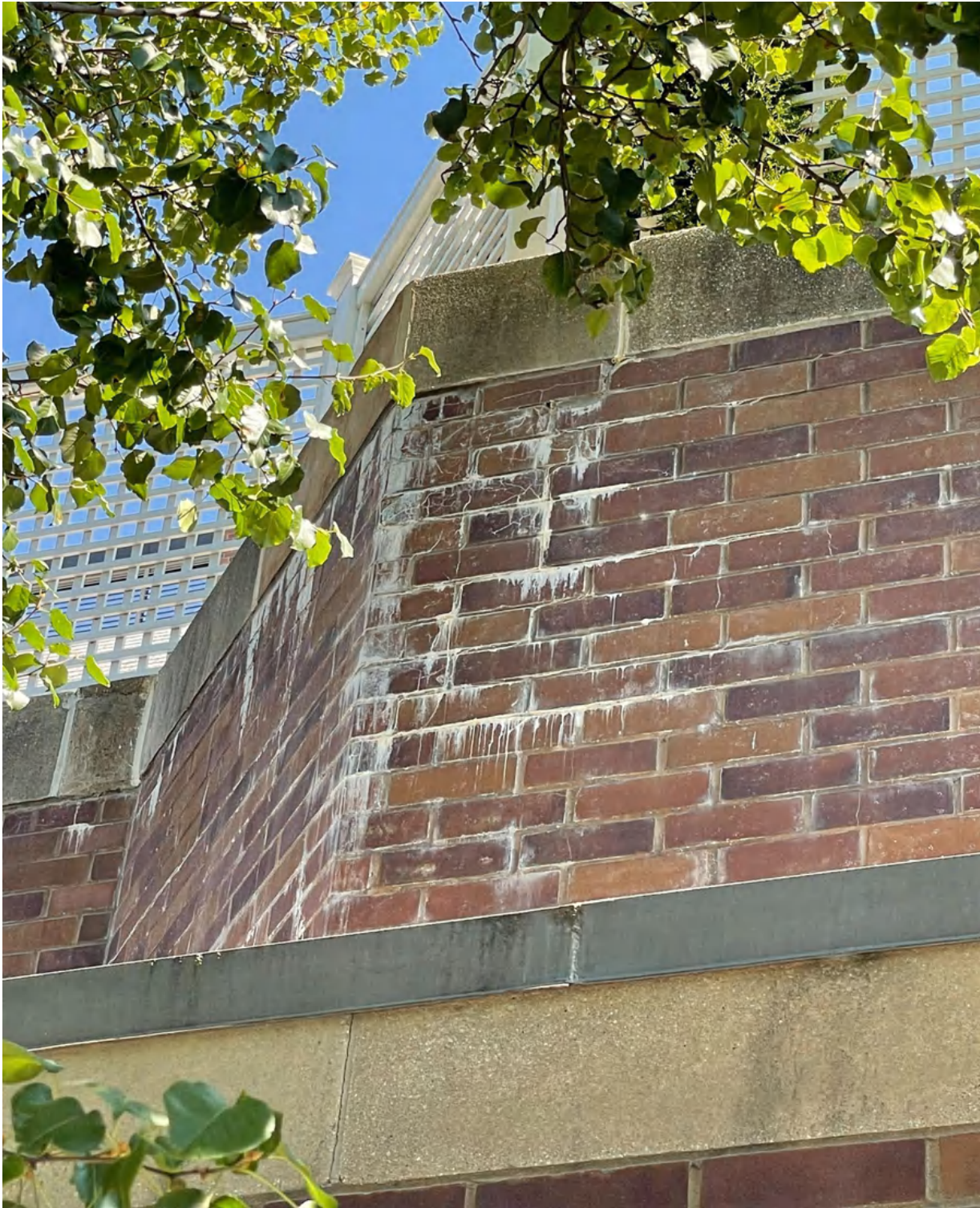
Photo 19: areas of heavy carbonate and efflorescence staining on brick veneer wall, at the pool planter wall
