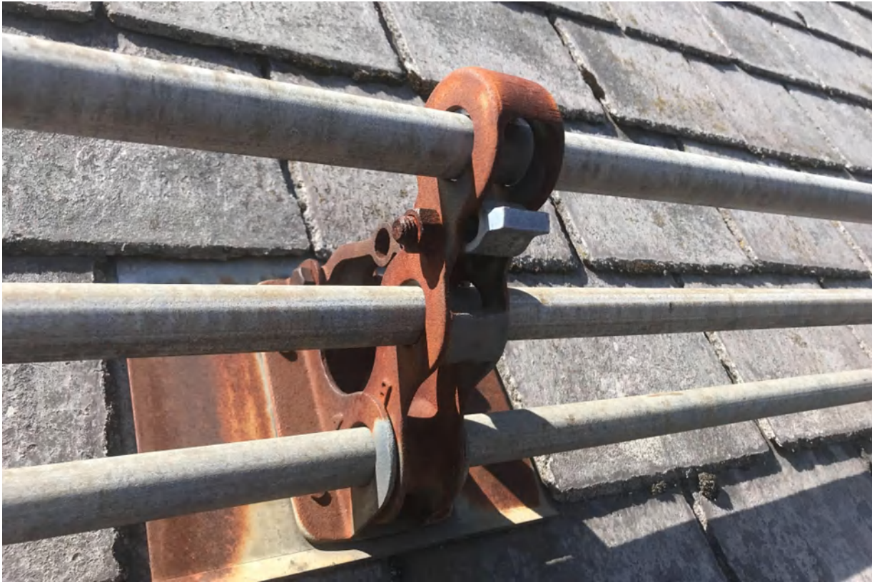
Photo 12: surface rust on the 3-pipe snow rail bracket (typical at majority of the brackets)
