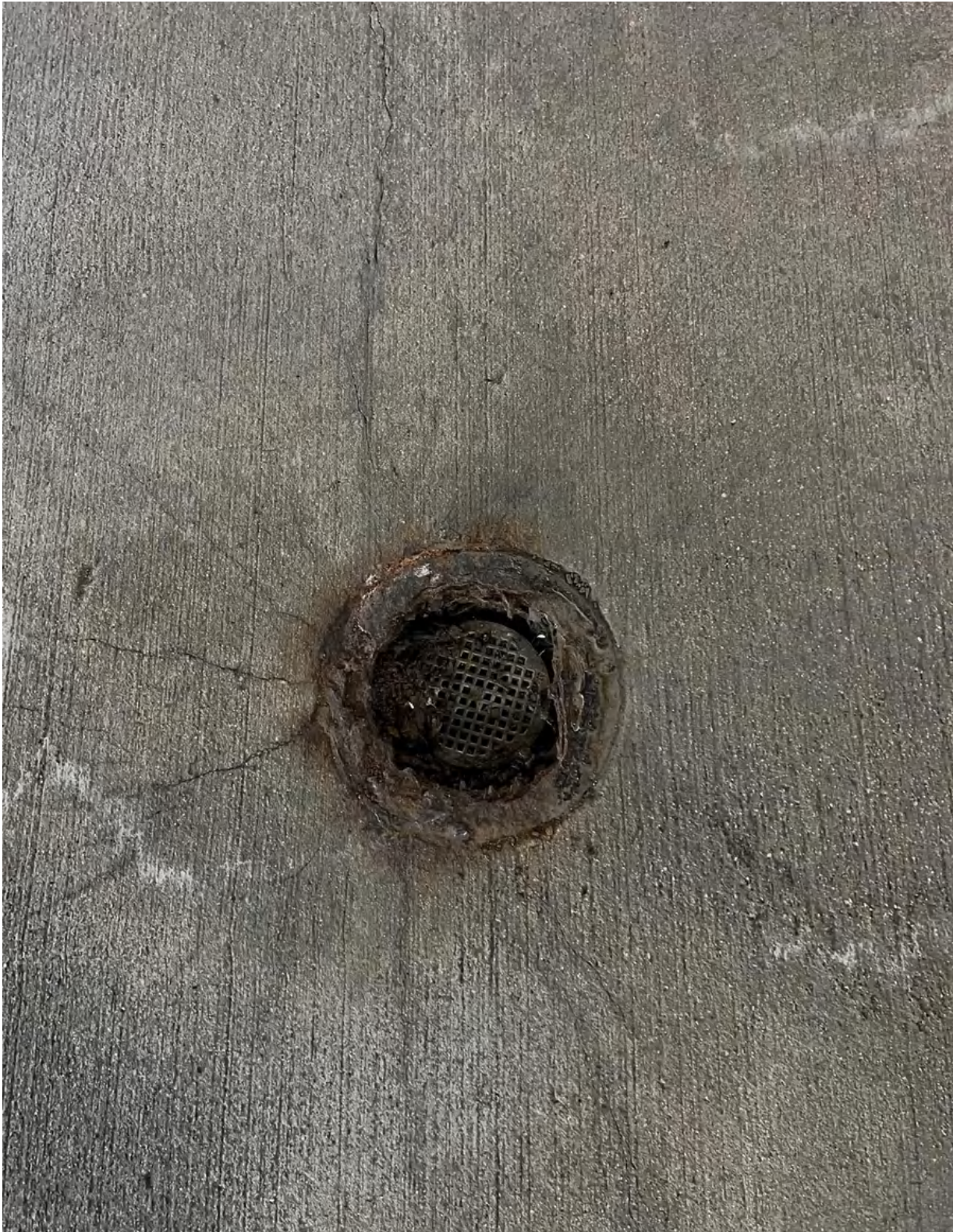
Photo 36: aged/damaged surface floor drain at the slab-on-grade floor slab
