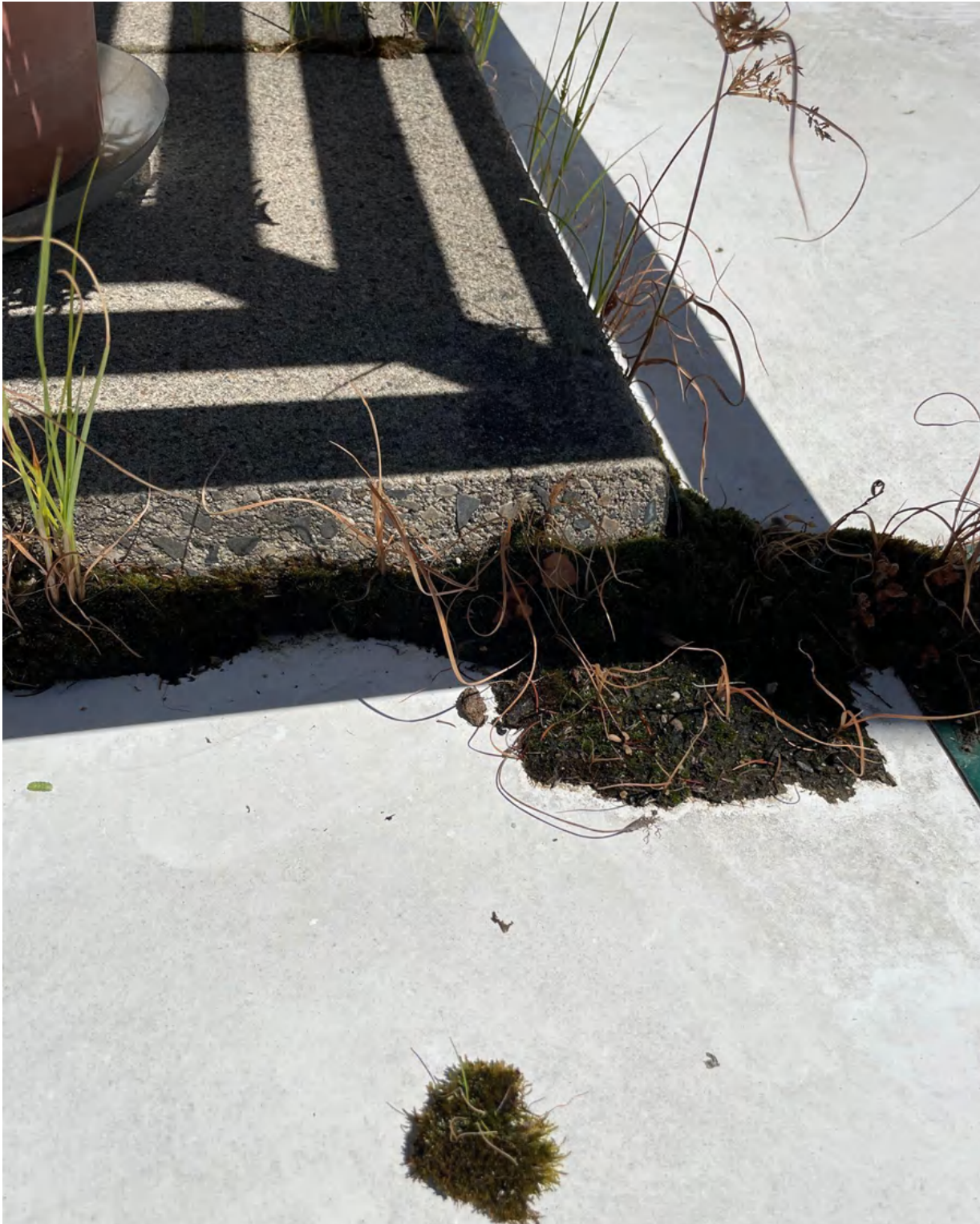
Photo 7: organic growth at perimeter areas of balcony precast pavers
