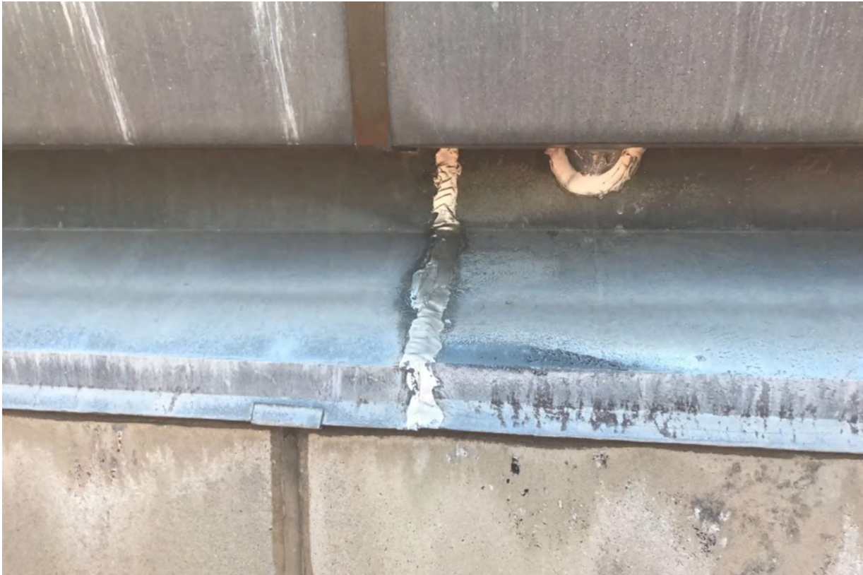
Photo 11: repaired solder joint in the copper, continuous transition cap flashing
