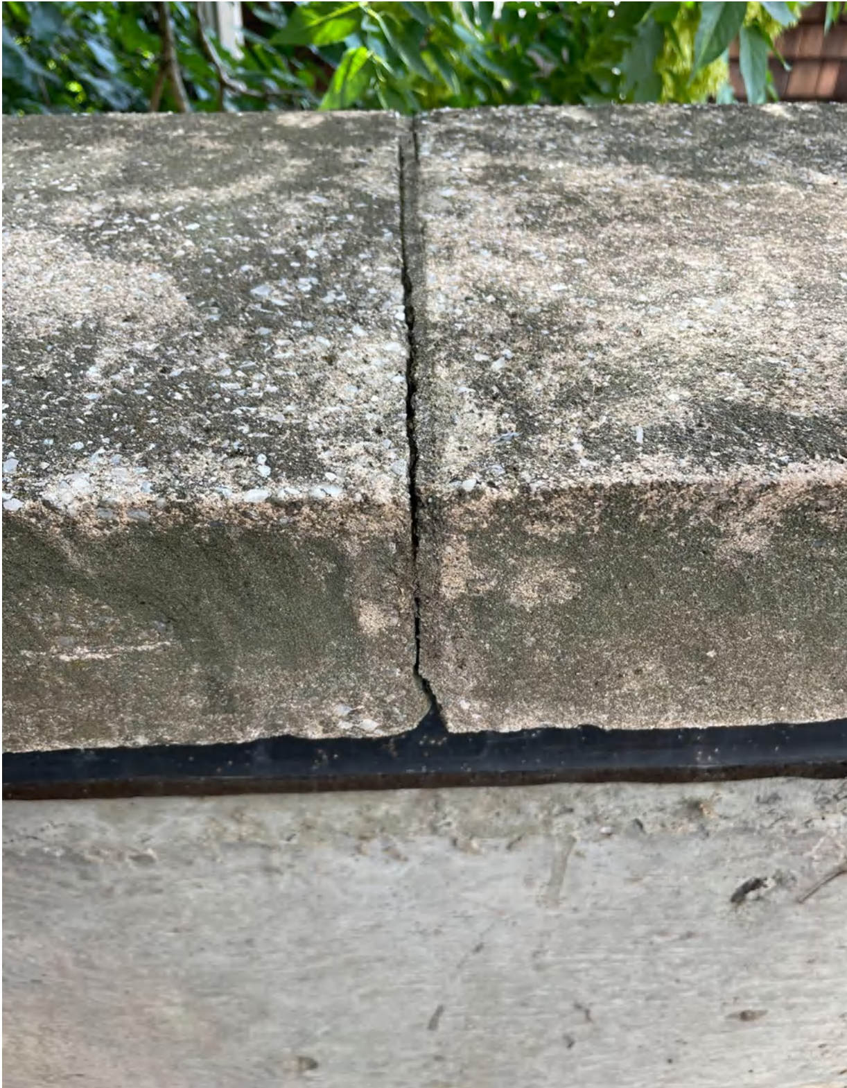
Photo 45: bond failure/cracking mortar joint between cast stone wall caps
