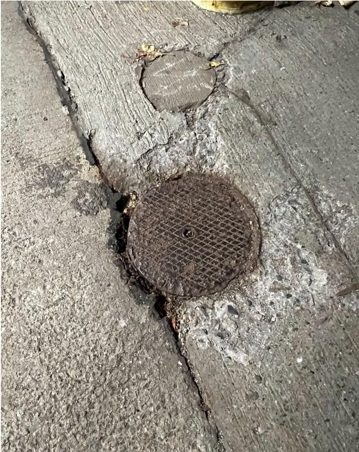
Photo 32: heavily rusted floor metal cap & concrete cracking/spalling
