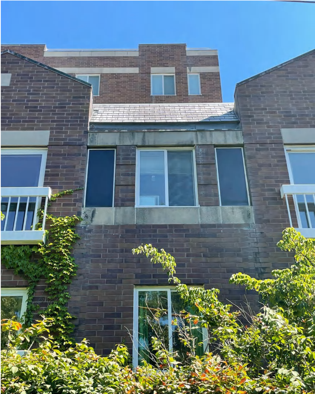
Photo 20: staining on brick veneer wall and cast stones directly below mansard roof edge/dormer rising wall interface areas - roof edge without gutters
