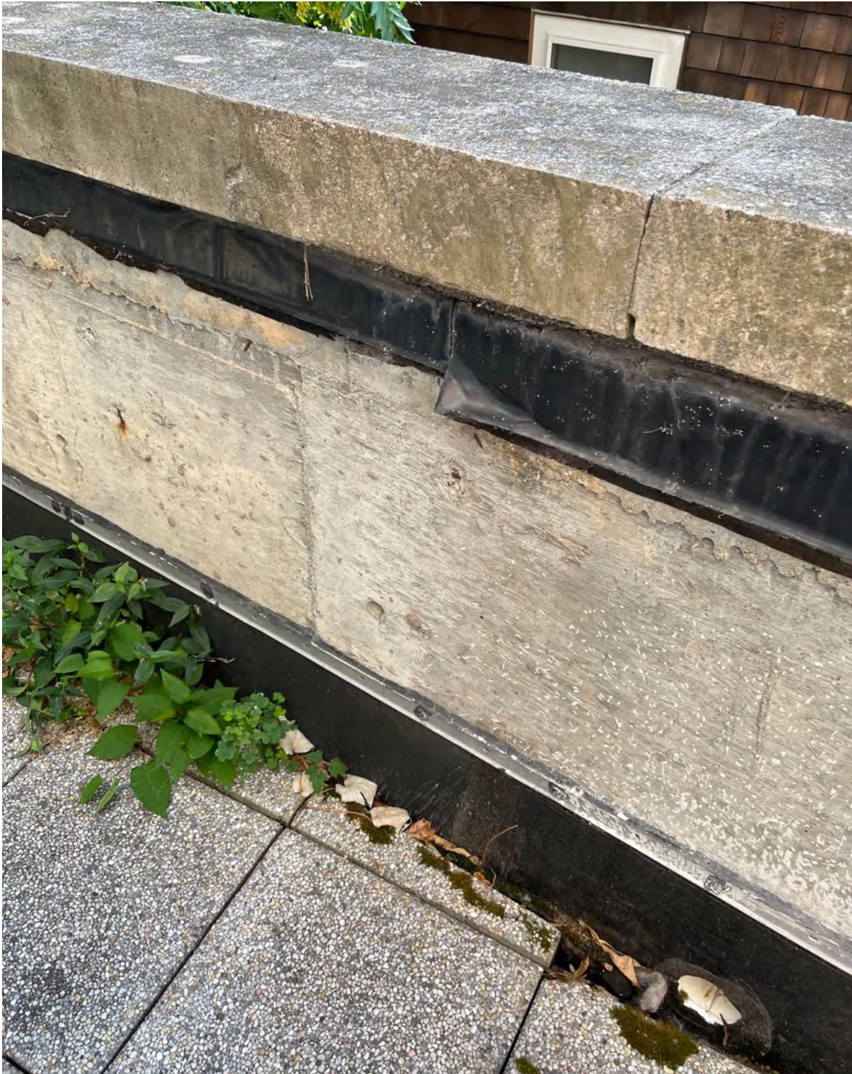
Photo 44: uncoated/bare concrete with cracking and unadhered rubberized asphalt sheet flashing with open seams used as wall cap flashing
