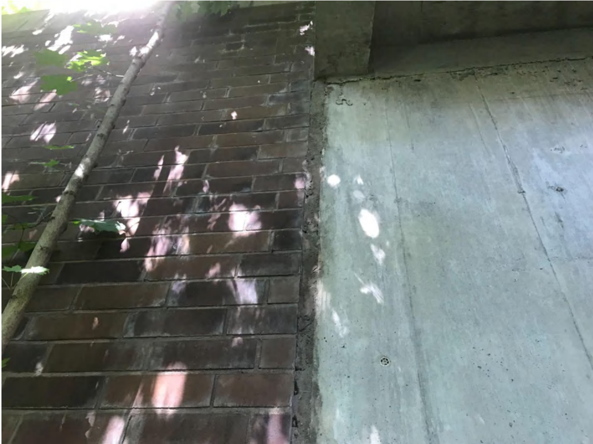
Photo 25: failing mortar joint at transition of brick veneer and concrete wall the east elevation
