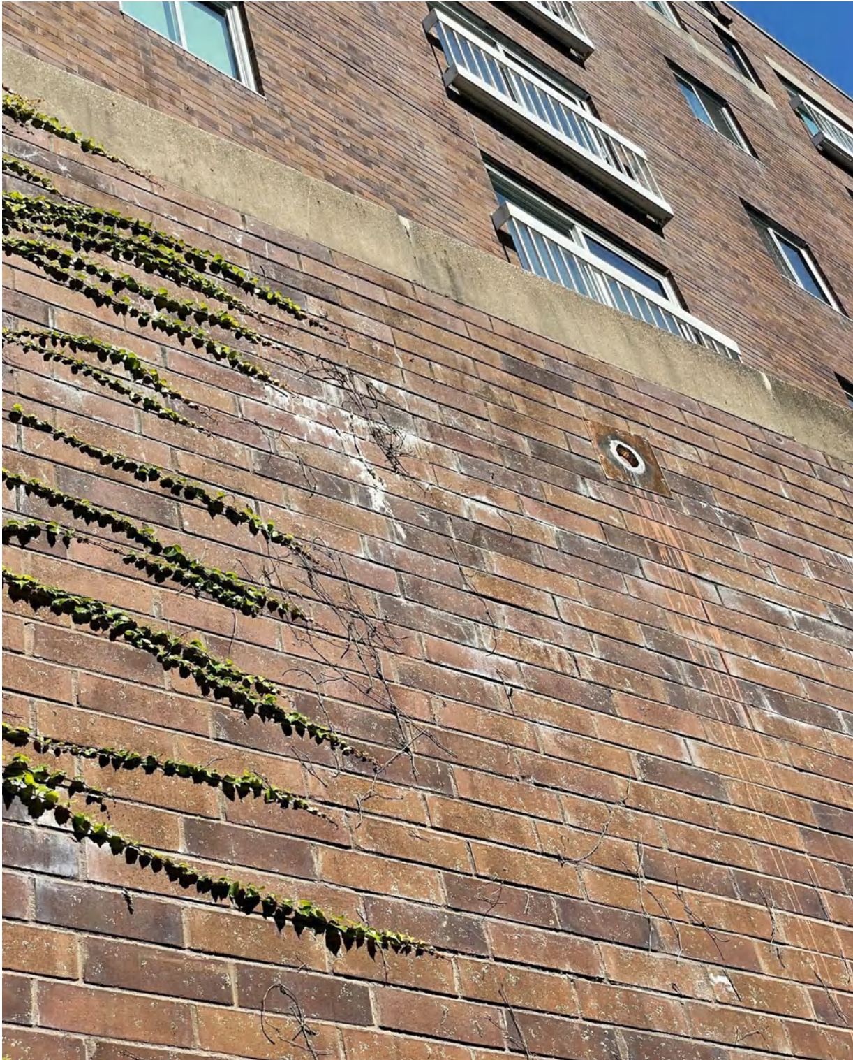
Photo 17: residue and staining on brick veneer wall surface adjacent to copper thru-wall scupper
