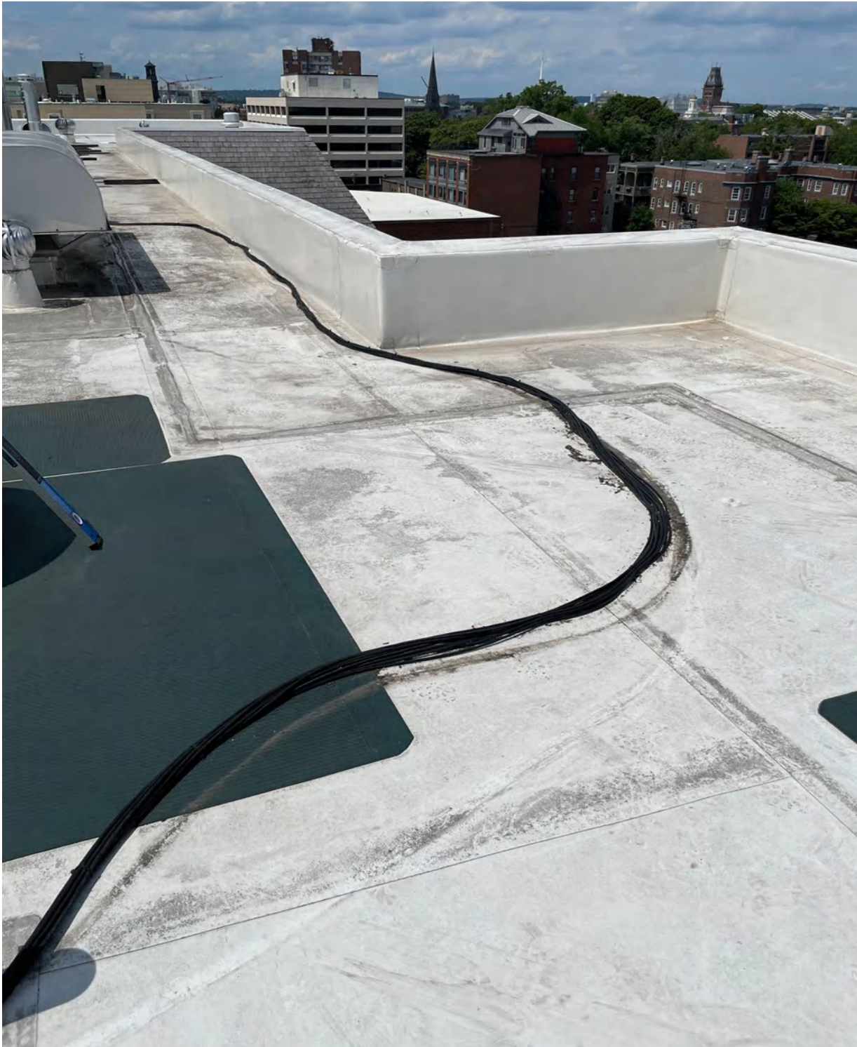
Photo 3: computer/data cabling laying directly on roof membrane surface (unattached)
