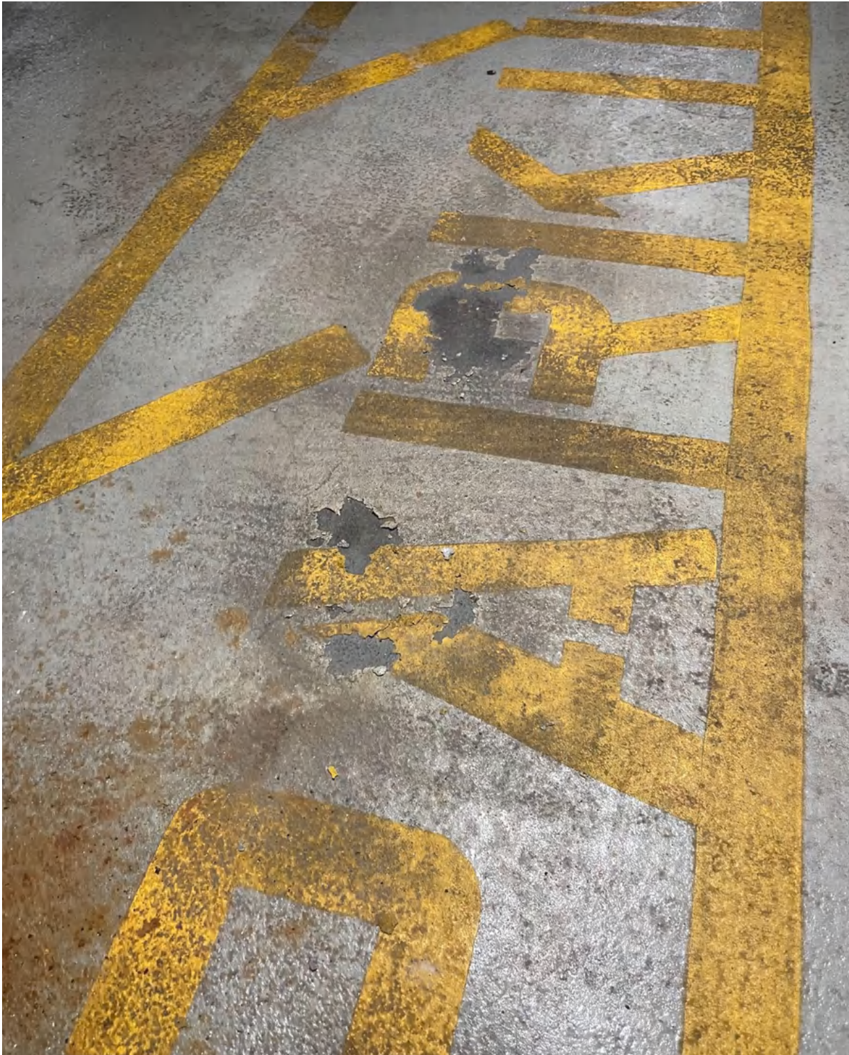
Photo 38: worn out/delaminated urethane traffic coating at upper level garage parking stall
