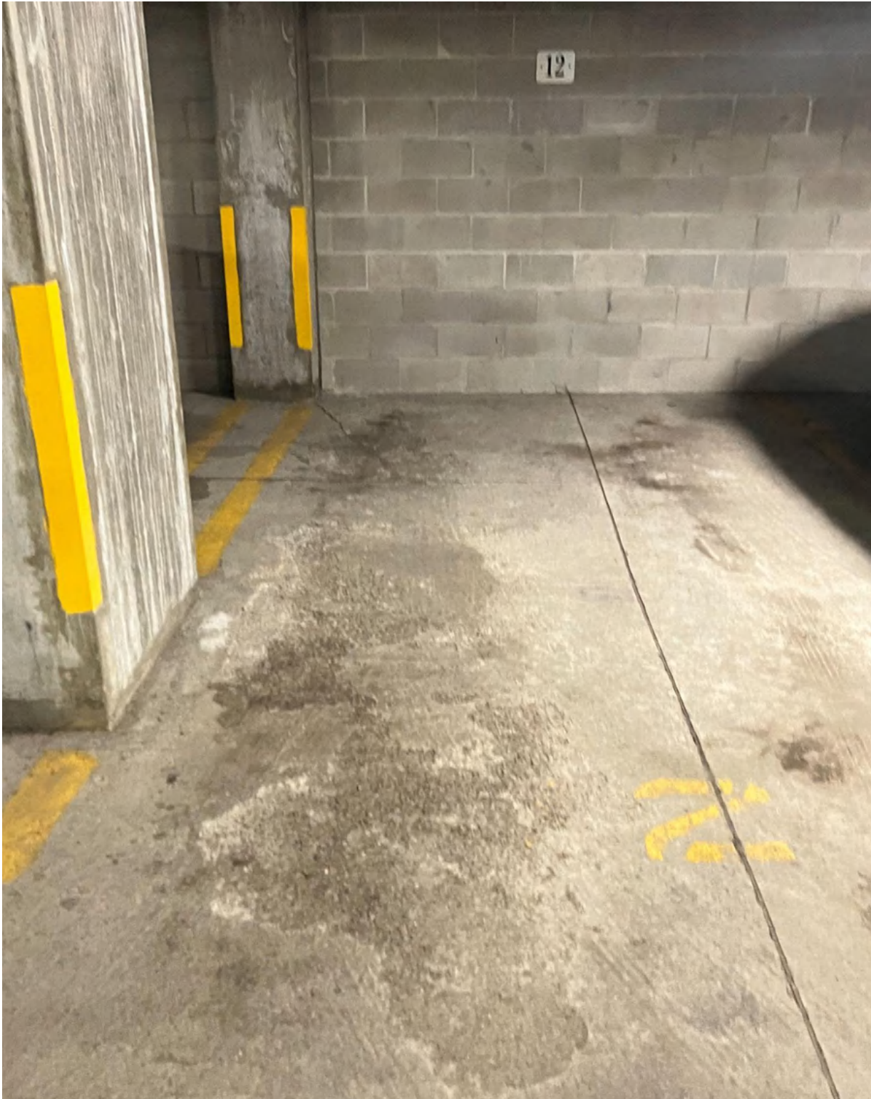
Photo 30: shallow concrete surface delamination at lower level garage parking stall
