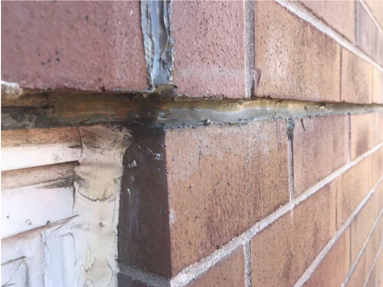
Photo 27: sealed weep hole at bedroom window header and relieving angle at 5th floor north elevation at unit #501
