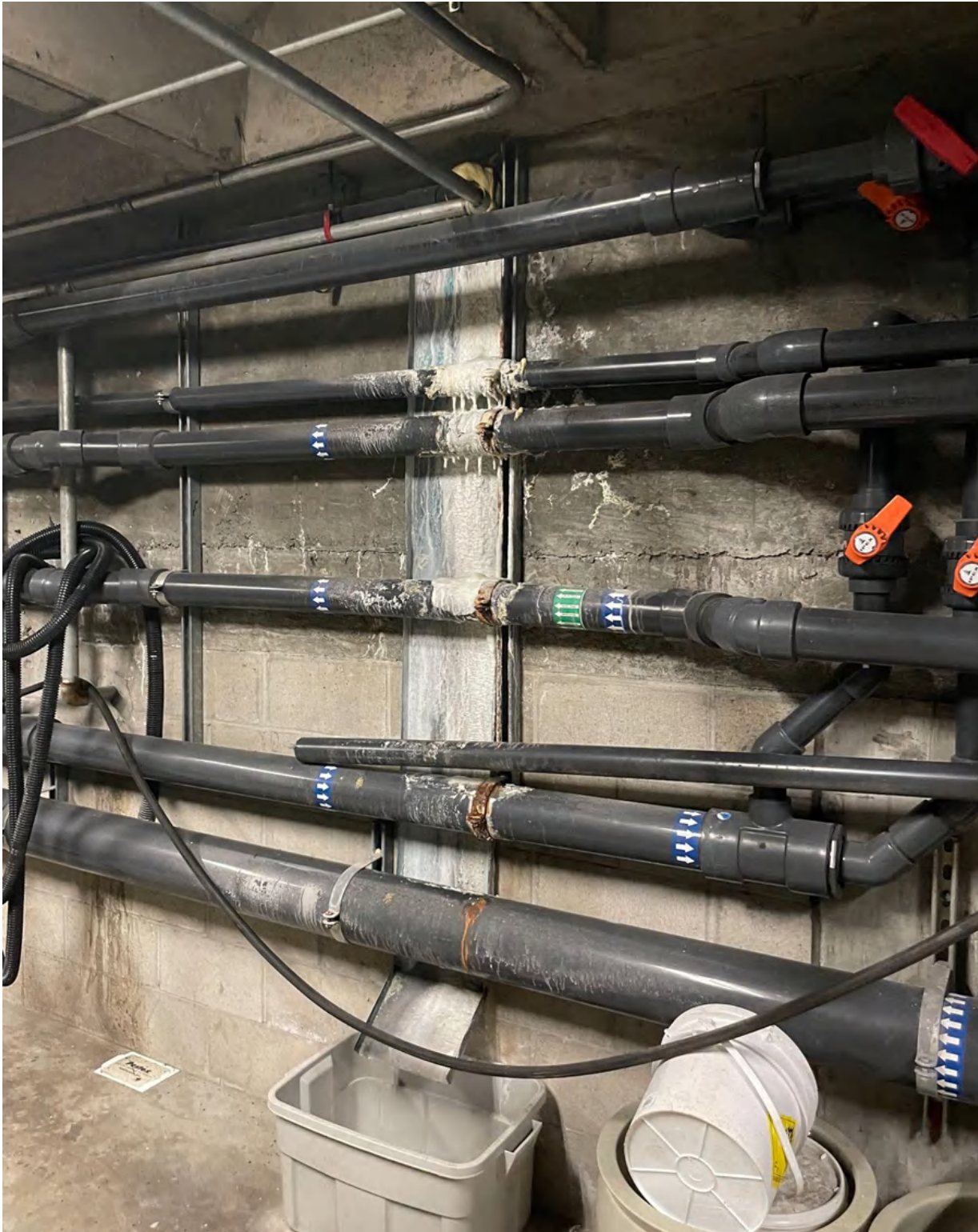
Photo 46: heavy carbonate staining on concrete pool wall and leak diverters attached to the wall directing active leak to collection bucket
