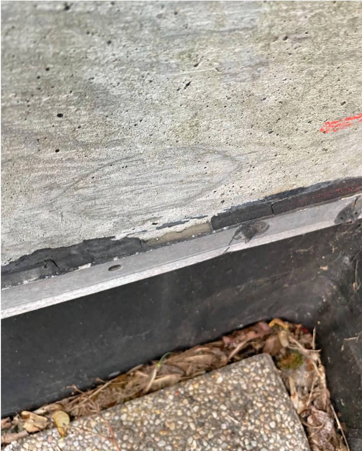
Photo 43: failed sealant at continuous aluminum termination bar (without counterflashing)
