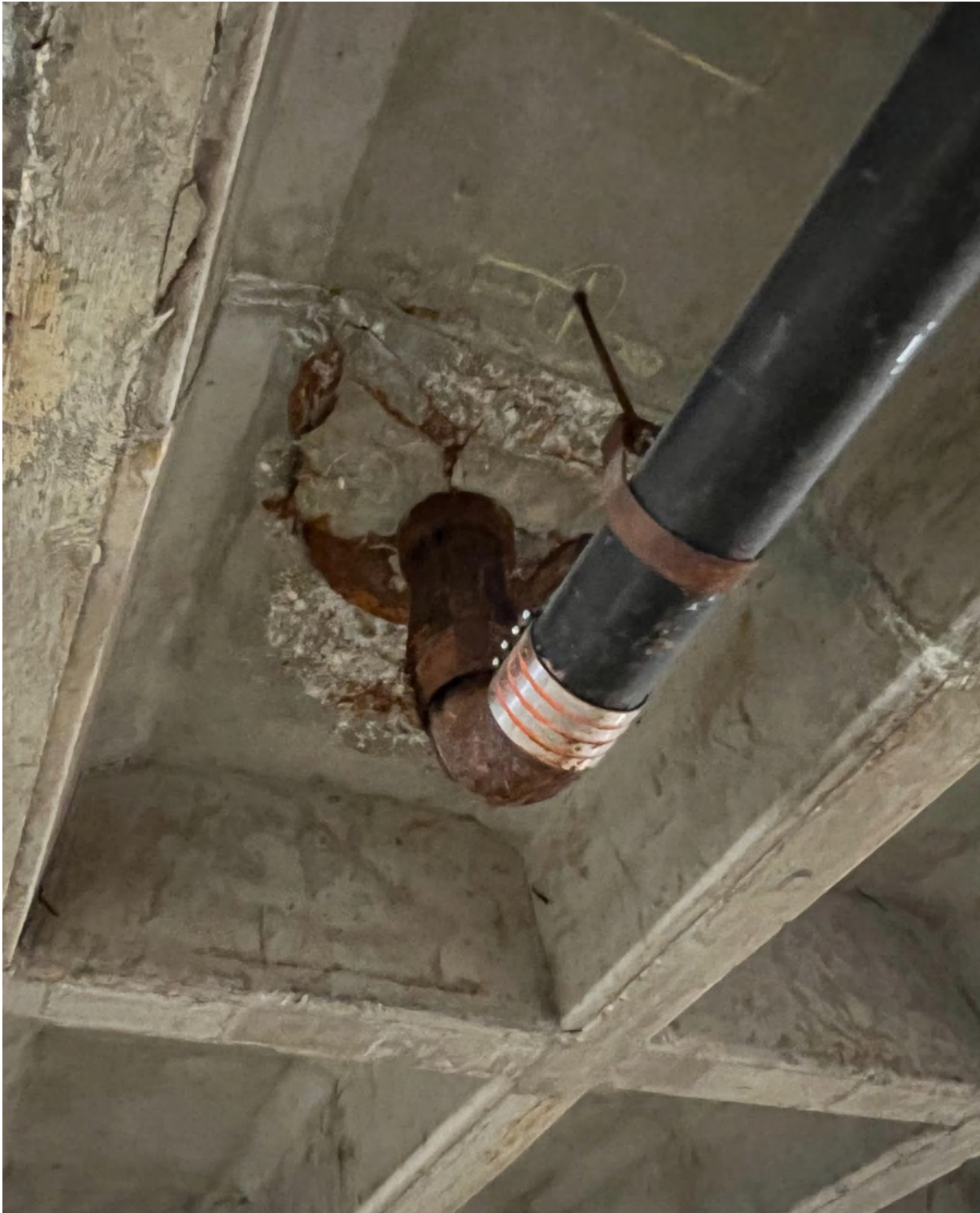
Photo 33: concrete damage consisting of spalling and cracking around upper level garage floor drain - Fall hazard to recieve “make-safe” action
