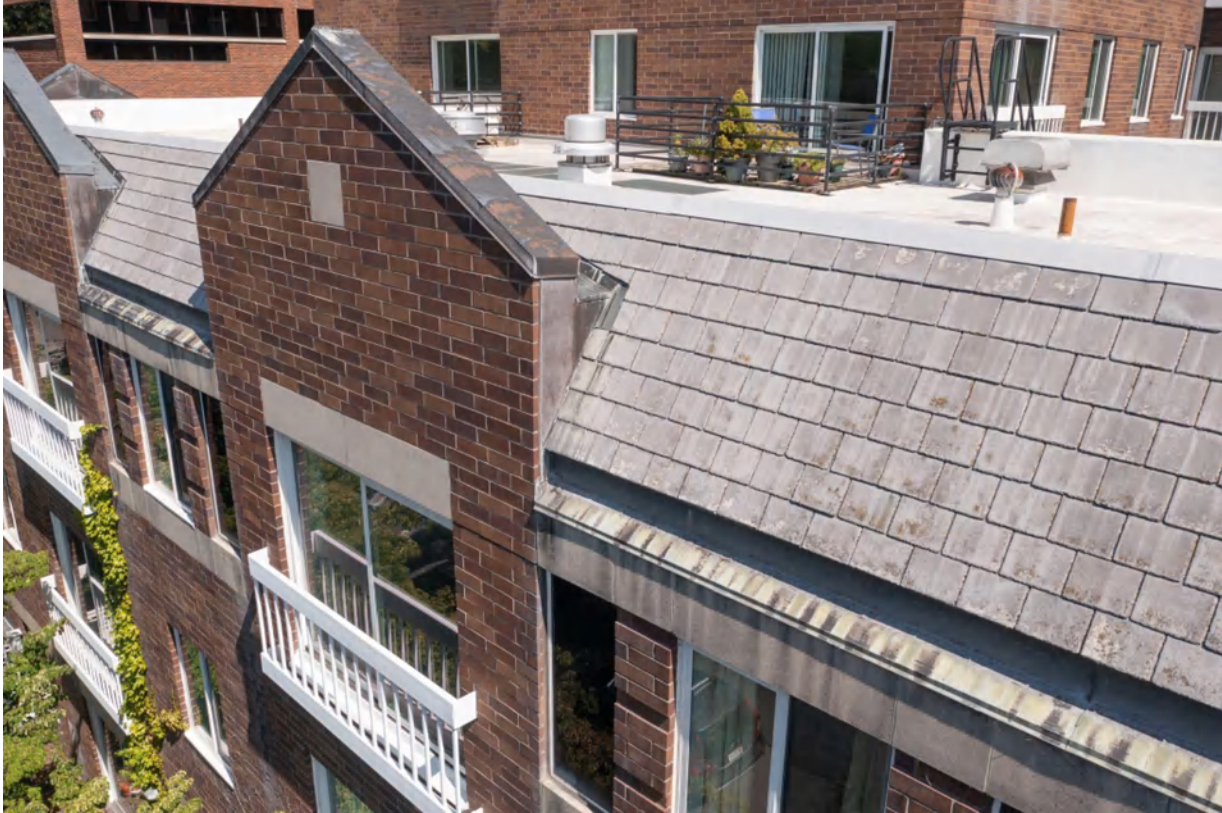
Photo 14: no snow rails, gutters or “kick-out” flashing at the mansard style, steep sloped roof on the south elevation
