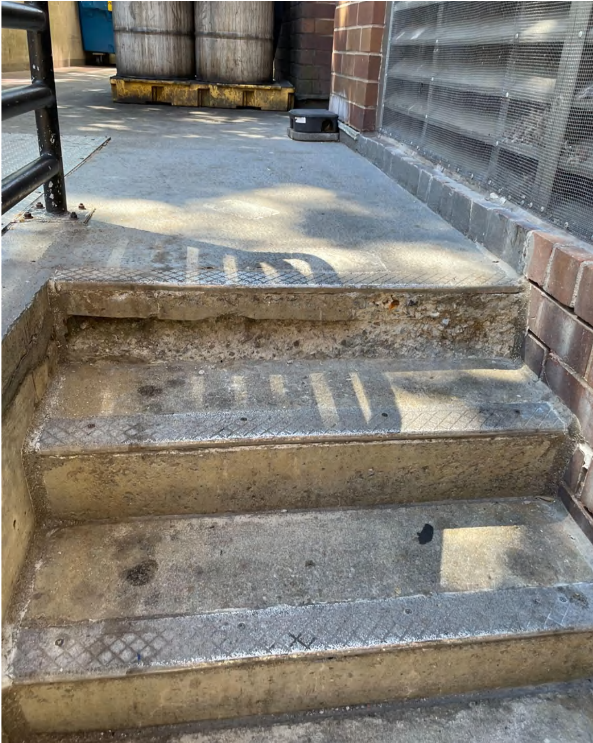
Photo 18: spalled concrete at loading dock stairs
