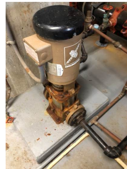
The ageing 2-horsepower fire-suppression system jockey pump shows signs of leaking and corrosion at its flange and base.
