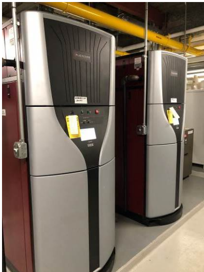
View of the RBI Flexcore condensing boilers, each with an input rating of 1500-MBH serving the two-pipe fan coil unit system.
