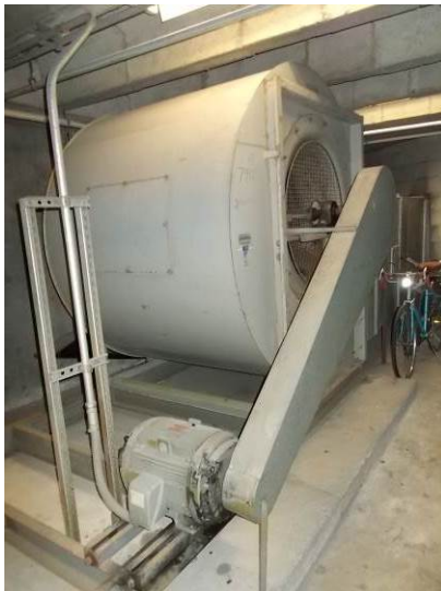
View of one of four garage ventilation and exhaust fan motors.
