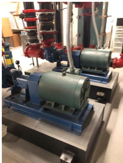
View of the Leeson WattSaver 30-hp, base-mounted service loop pumps.
