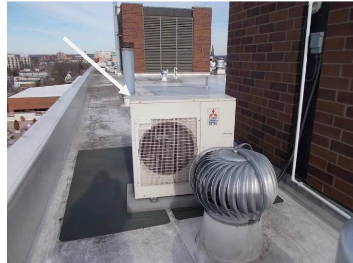
The elevator penthouses are heated / cooled by split system heat pumps.
