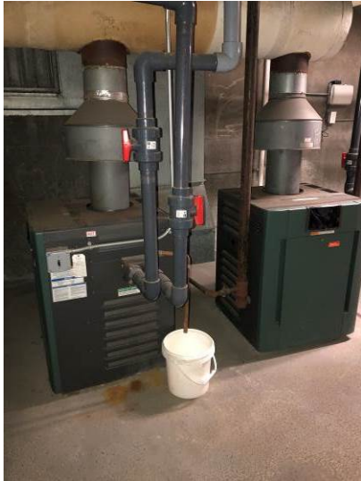
RayPak 399-MBH natural gas-fired boilers used to heat the pool water, both were installed in 2008.
