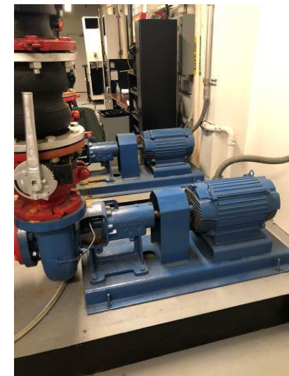
View of the 20-hp, base-mounted cooling tower loop circulating pumps.
