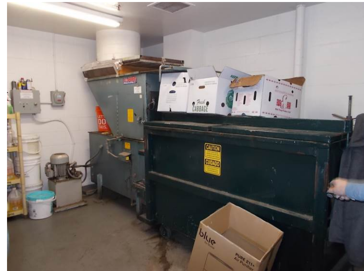
View of the chut-fed, hydraulic compactor and two-cubic yard rolling trash containers.
