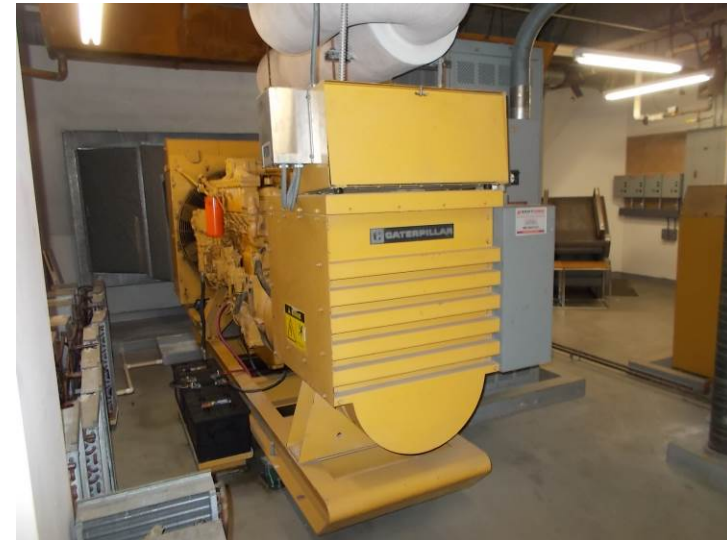
The 300 kW Caterpillar diesel-fired generator is located on the 7th floor level.
