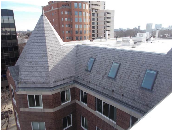
View of the fiber-cement faux-slate shingles on the mansard.
