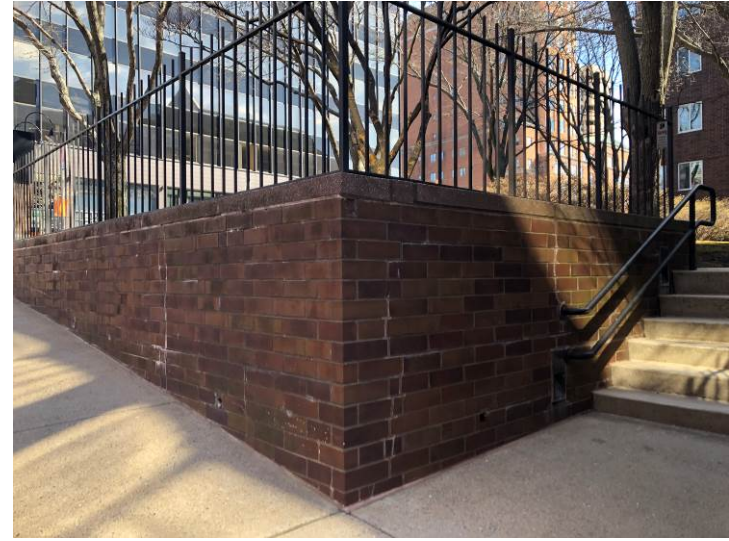
The Bay Street side of the front park has brick retaining walls and recently replaced concrete stairs.
