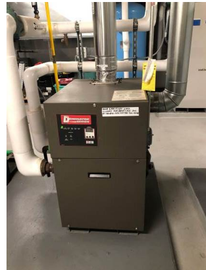
The RBI Dominator 300-MBH boiler was installed in 2016 to produce hydronic heat for the boiler, storage, and generator rooms.
