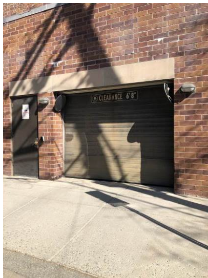
The townhouse garage has a single fiberglass overhead door; access is at the rear of the building
