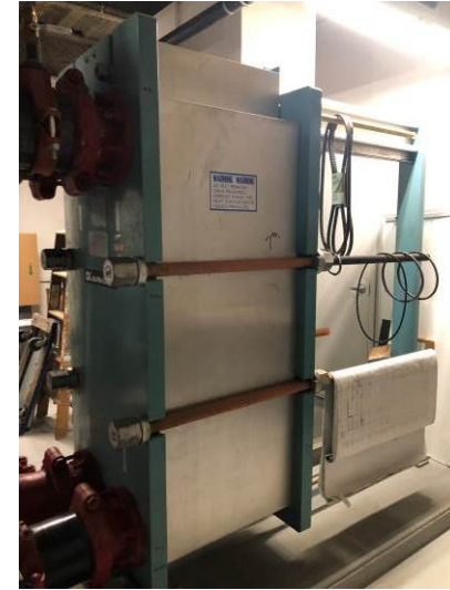
View of the Alfa-Laval A15-BFG, 4600 sf, 150 PSI, plate and frame heat exchanger believed to be original to the construction of the building.
