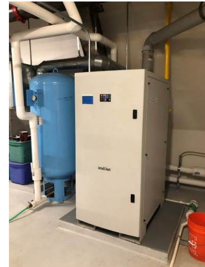
View of one of two Intellihot, natural gas-fired, 1001-MBH domestic hot water boilers. Both boilers were installed in 2016 and are in good current condition.
