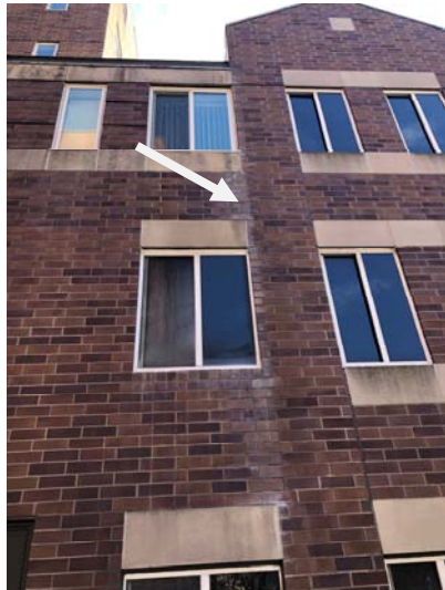
Visible efflorescence noted at various elevations of the building.
