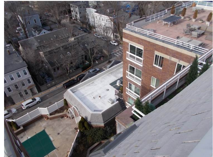
Adhered reflecting polyvinyl chloride (PVC) membrane on the 2nd floor roof installed in 2007.
