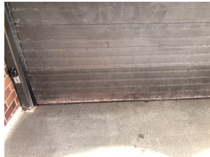
Rusting and surface deterioration was observed on many of the garage doors.
