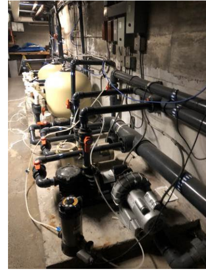
View of the various pool and spa mechanicals including sand filters, chlorinators, and pumps.
