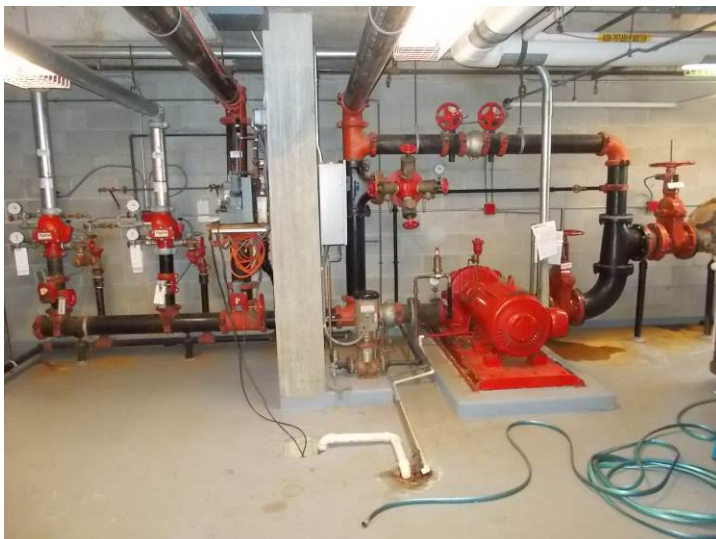
View of the Lincoln wet-pipe fire suppression system 75-horsepower electric fire pump (on the right); maintained, tested, and serviced on a regular basis.
