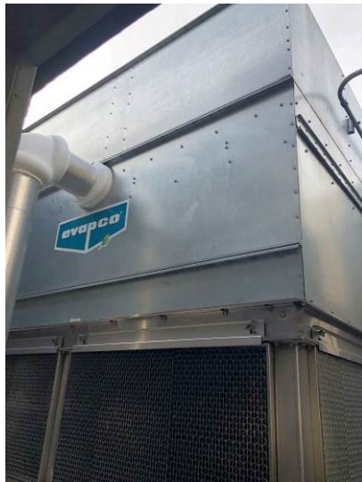
View of the Evapco AT-112-612, induced-draft, counterflow cooling tower located on the roof.
