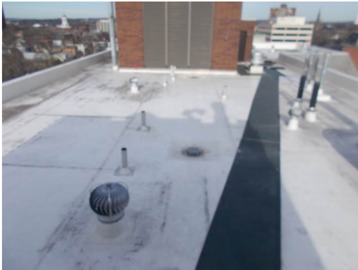
View of the Sarnafil PVC membrane roof installed in 2009.
