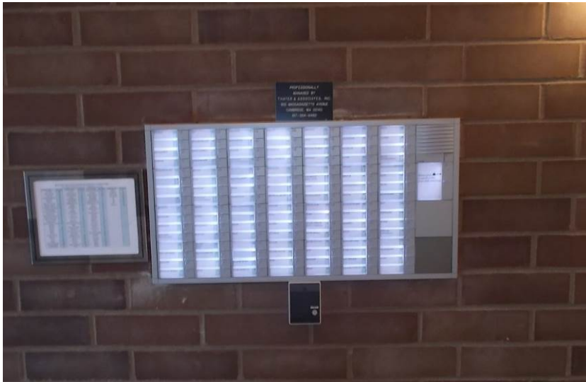
View of the door buzzer/intercom panel located at the front entrance vestibule.
