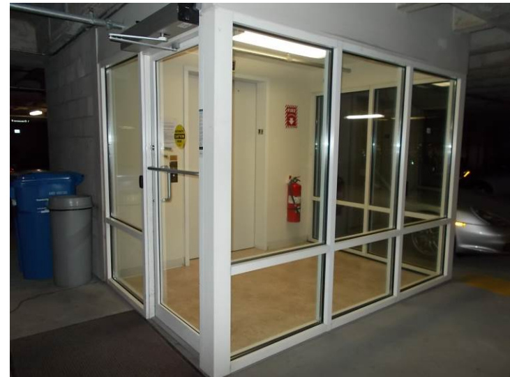
View of one of four garage vestibules. All vestibules have power door openers and fob entry panels.
