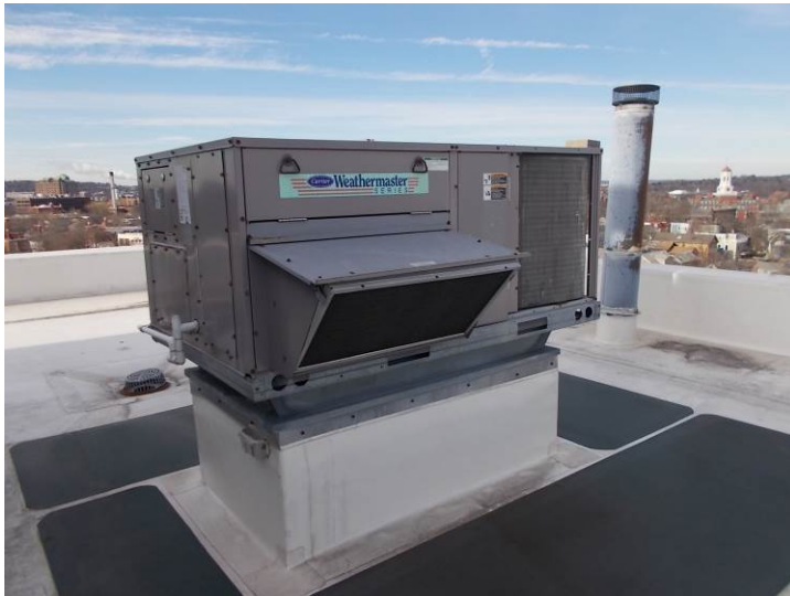
One of two, Carrier WeatherMaster, 4-ton, single-package rooftop units serving the common hallways.
