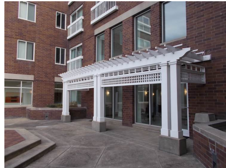
An Azek PVC framed pergola, installed in 2009, frames the rear lobby entrance.
