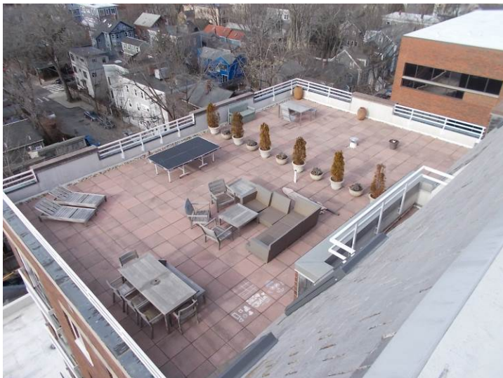
The southwest private terraces had new EPDM membrane installed in 2020 and the concrete pavers were reused/replaced.
