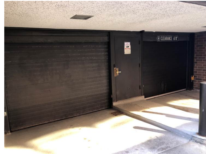
The upper and lower garage each have a pair of fiberglass segmented-panel overhead doors with power door operators.
