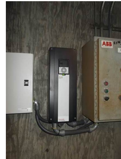
New Honeywell VFD's were installed in 2017 on all four of the garage ventilation fans.
