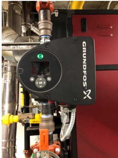
Grundfos Magna3 stainless steel circulator pumps circulate boiler water.
