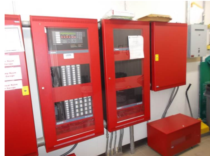
View of the Simplex 4100U fully addressable fire alarm control panel with command center.
