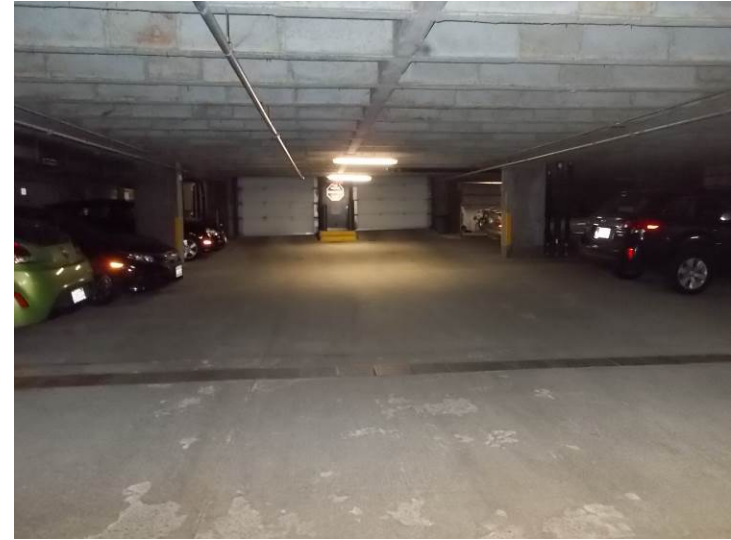
The lower garage concrete deck exhibits areas of surface deterioration.
