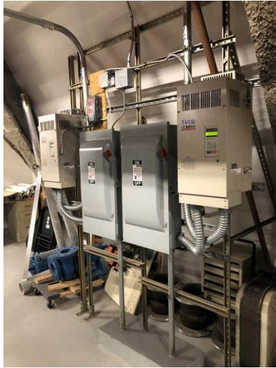
Teco MA7200 variable frequency drives (VFD) were installed in 2014 on each service loop pump.
