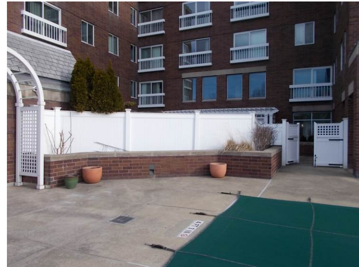
View of the Azek PVC fencing, arbor, and gate which were installed in 2012.
