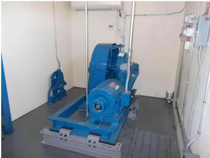
View of the west elevator Imperial Electric 25-horsepower traction machine located in the elevator penthouse. The east elevator is similar.
