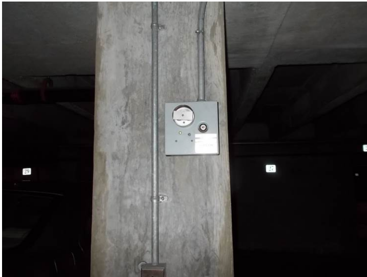
View of a typical wall-mounted CO sensors located throughout the garage. The system activates the four intake and exhaust fans.
