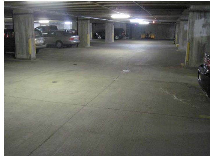
The lower garage currently has no epoxy concrete deck surface coating.
