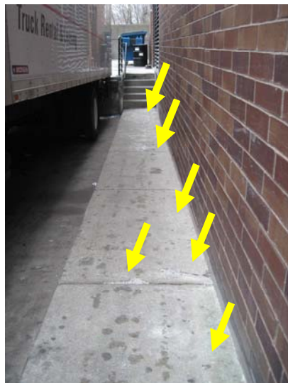
View of the loading and trash removal dock at the building east elevation. Note general surface deterioration and cracking visible at several locations along the walkway.
