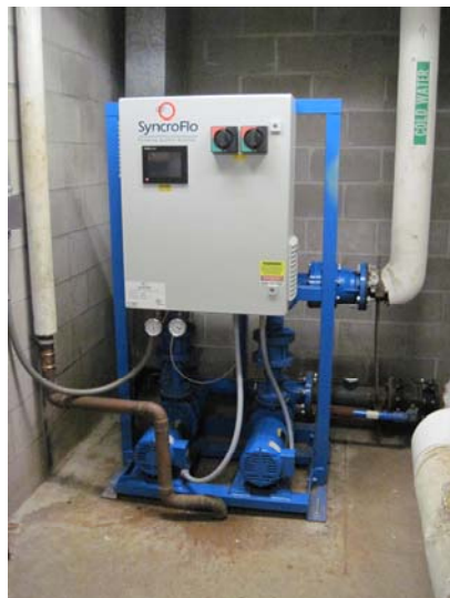
View of the SyncroFlo cold water booster system with dual Baldor 5-horsepower pumps.
