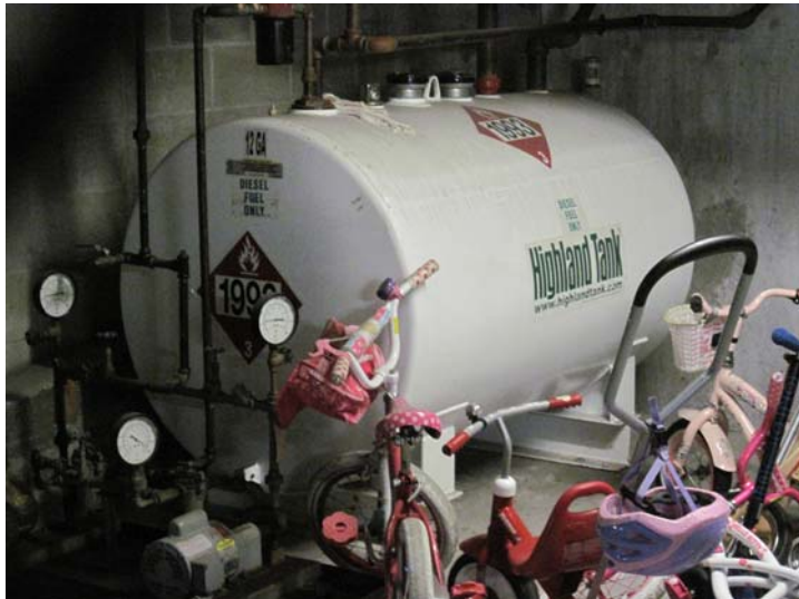
The 450-gallon generator diesel fuel storage tank was newly installed in the parking garage in 2013.
