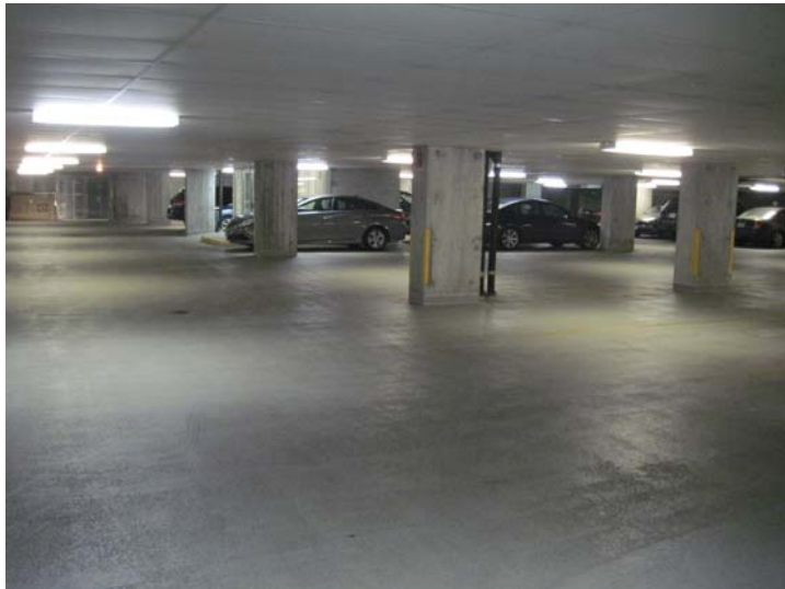
The upper garage features a suspended acoustic tile ceiling and epoxy deck surface coating.
