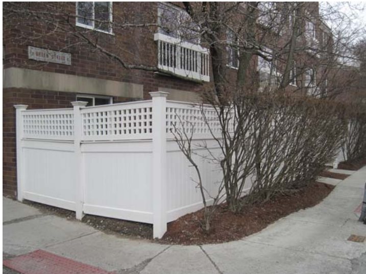
The townhouse-style units at the rear (Green Street) elevation feature low-maintenance Azek PVC privacy screen fence enclosures, all newly installed in 2012
