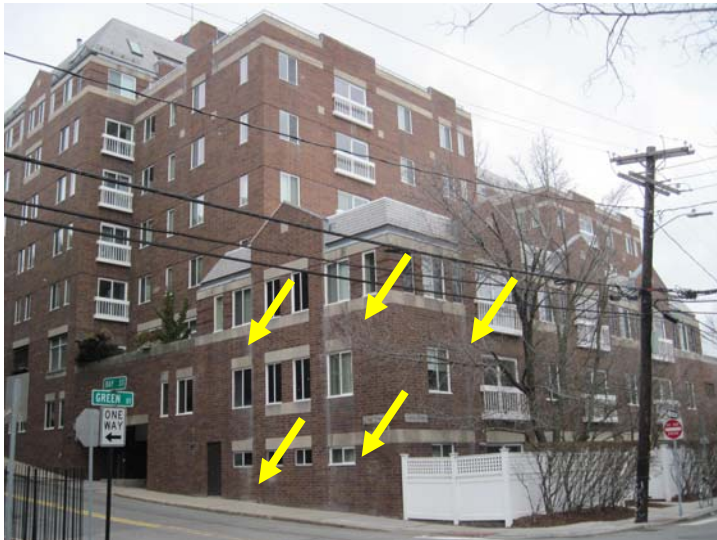
View of the rear (south) Green Street elevation. Note visible efflorescence at southwest corner.
