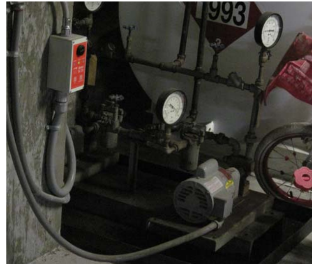
A dual-pump fuel delivery system transfers the fuel up to the 7 th floor generator room day tank.
