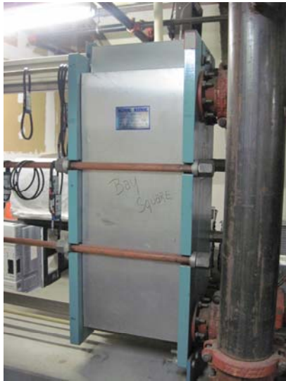
The service loop is warmed by the boiler water or cooled by the cooling tower water via this Alfa-Laval A15-BFG, 4600 sf, 150 PSI, plate and frame heat exchanger.
