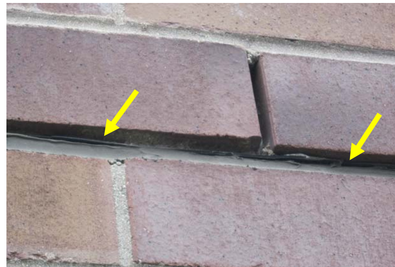
Close-up of control joint cohesion failure.
