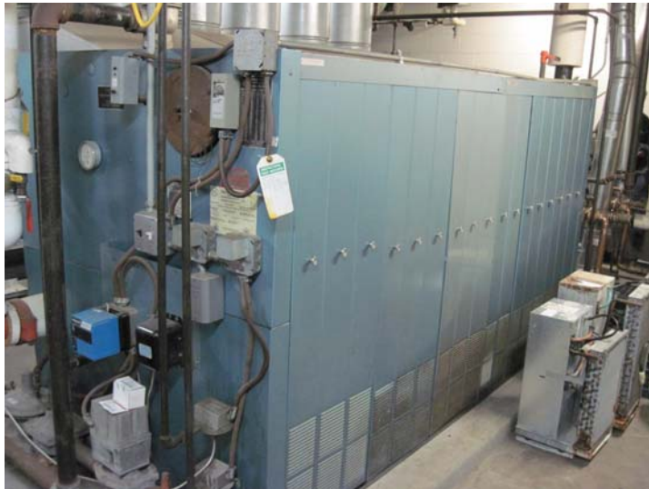
View of the 3,825 MBH, H.B. Smith sectional cast-iron natural gas-fired hot water boiler serving the two-pipe fan coil unit system.
