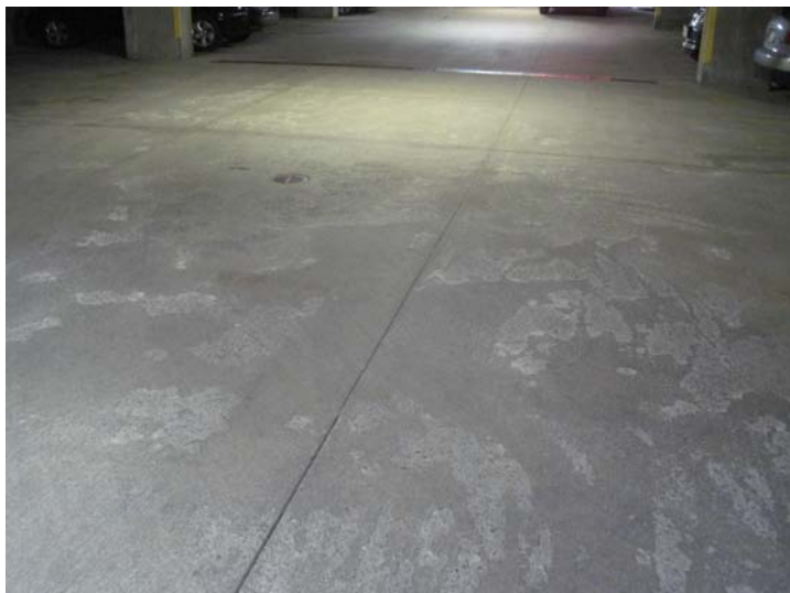
The lower garage concrete deck exhibits areas of surface deterioration. In need of repair, resurfacing, and an epoxy deck coating.
