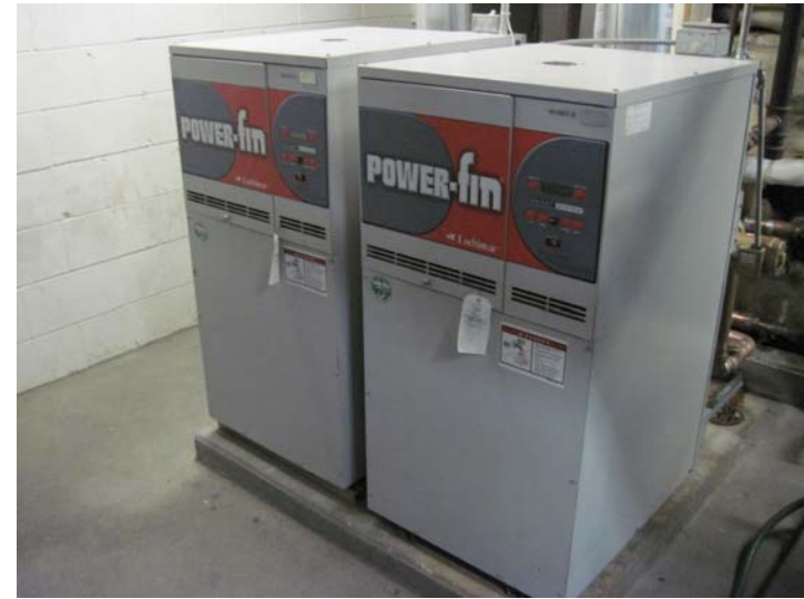
The building domestic hot water is created by this pair of dedicated Power-Fin 500 MBH (87% AFUE) natural gas-fired DHW boilers.
