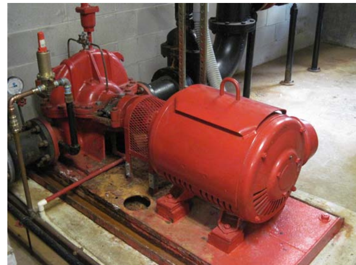
View of the Lincoln wet-pipe fire suppression system 75-horsepower electric fire pump; maintained, tested, and serviced on a regular basis.
