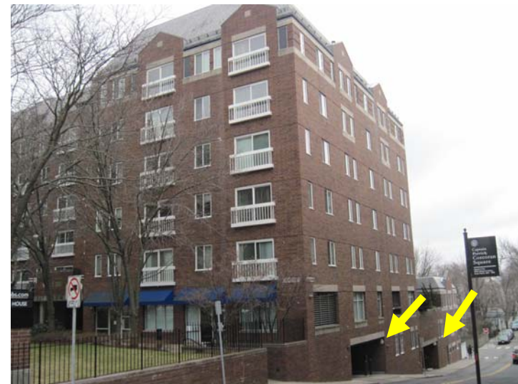
View of the west (Bay Street) elevation. Note upper and lower garage entrance/exits. Balcony railings were all coated in 2010 with a RhinoShield ceramic paint carrying a 25-year warranty.
