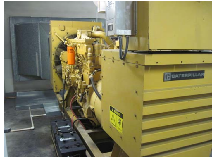
The 300 kW Caterpillar diesel-fired generator is interiorly located on the 7 th floor Mansard level.
