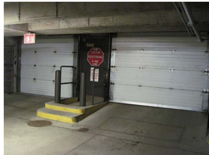
The upper and lower garage each feature powered fiberglass segmented-panel overhead vehicle entry and exit doors flanking a flush metal passage door.
