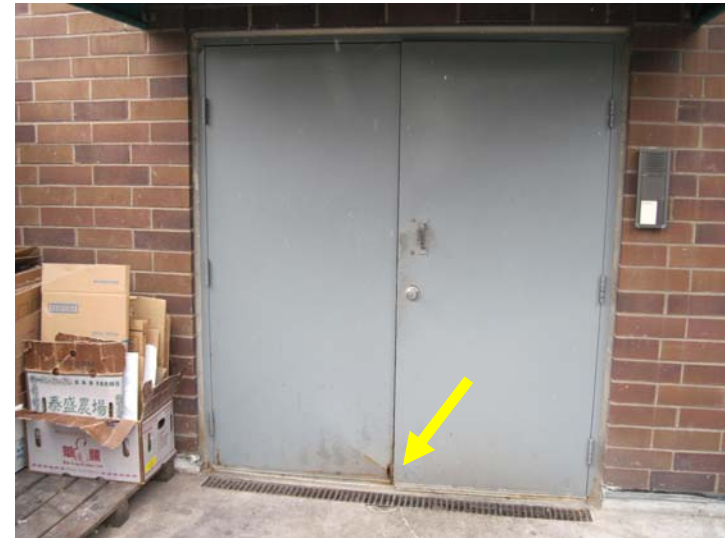
The aging loading dock flush metal service doors is corroding at the base and in need of replacement in the near term.
