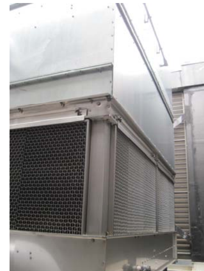
View of the Evapco induced draft, counterflow cooling tower. Newly installed in 2012.
