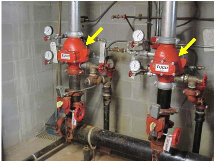
View of the new dry-valves installed in 2015.
