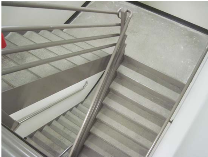
Egress stairwells feature painted walls and ceilings, painted steel stringers and railings, and concrete treads and landings.
