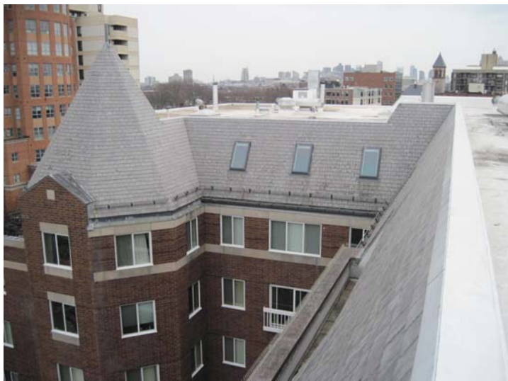
The steeply pitched Mansard level roof features faux-slate fiber-cement shingles.
