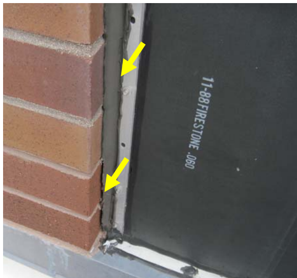
Door and control joint caulk exhibit age-related cohesion failure many locations. In need of replacing.
