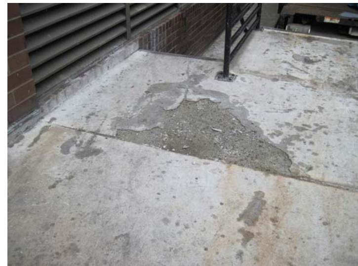
Sectional concrete deterioration and cracking is visible on the loading dock surface as well.
