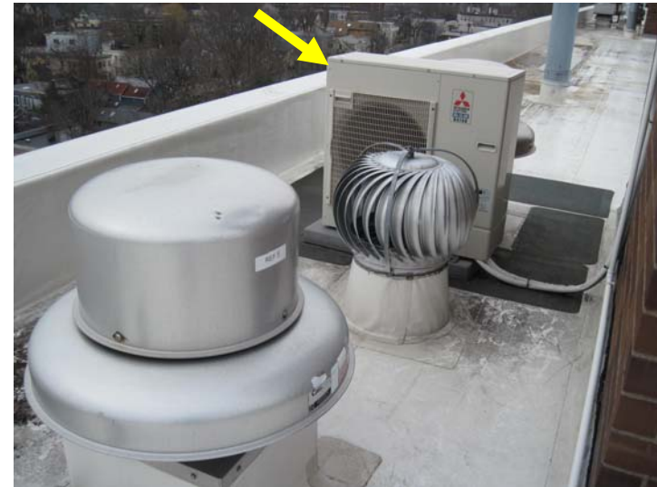
View of typical mushroom-type down-blast rooftop exhaust fans and the Mitsubishi 2-ton mini-split system heat pump (arrow) that heats and cools the east elevator machine room. The west elevator machine room is heated and cooled by a similar unit.
