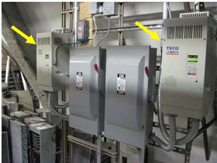
The service loop pumps are each controlled by a 40-hp Teco MA7200 variable frequency drive (VFD) which save energy, reduce wear and tear, and help extend the life of the pumps
