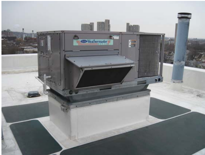
Two Carrier 4-ton, high-efficiency (SEER 13) single-package rooftop unit (RTU) that provide fresh and conditioned air to the hallways.
