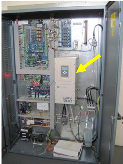
New solid state elevator controls with Magnatek HPV900 AC drives (arrow) were also installed in 2014.
