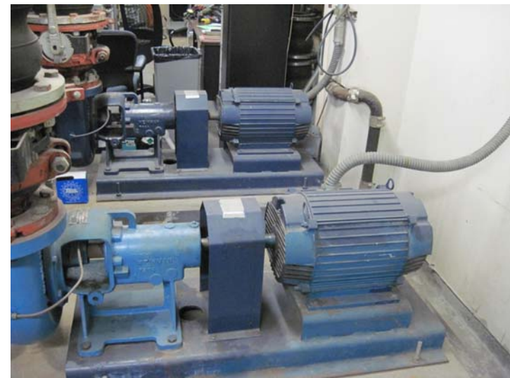
The cooling tower water is circulated by this pair of 20-hp base-mounted pumps.
