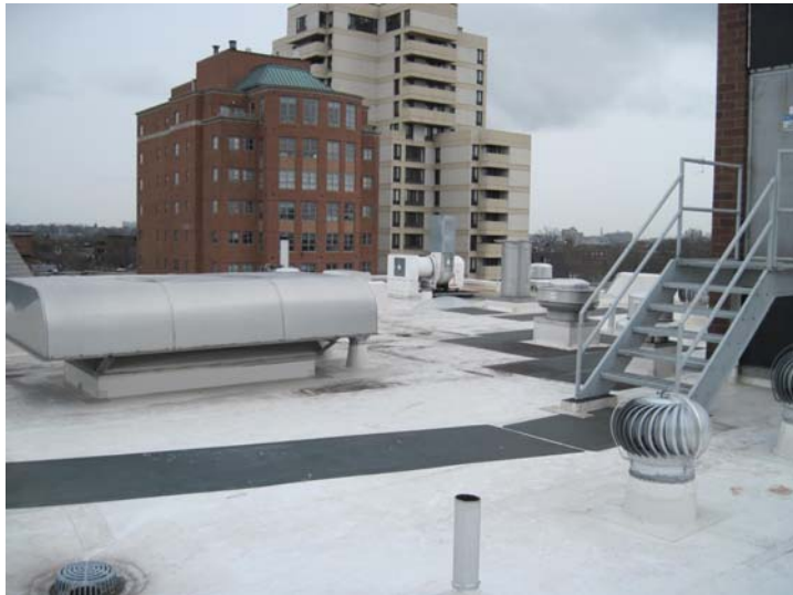
View of the Sarnafil PVC membrane roof and variety of exhaust and stairwell pressurization fans.
