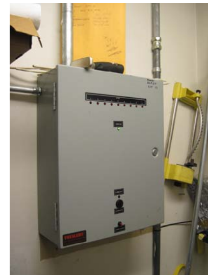
View of the parking garage ToxAlert carbon monoxide (CO) detection system control panel.
