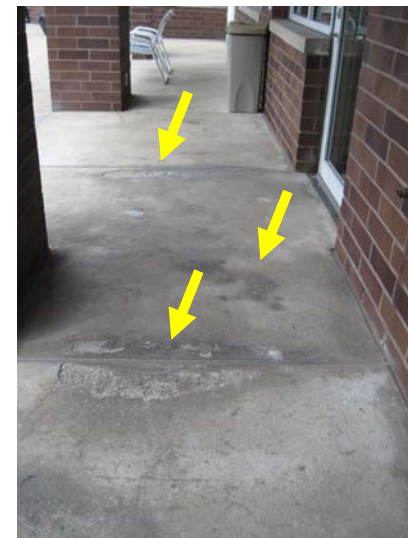
Sectional concrete surface deterioration is visible at the pool area and rear courtyard; in need of sectional repair/resurfacing.
