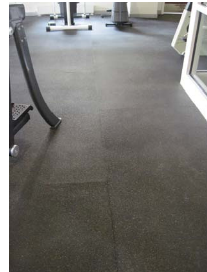
The fitness room rolled rubber flooring is showing signs of age and use related wear.
