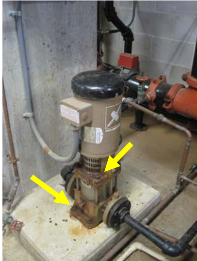
The ageing 2-horsepower fire-suppression system jockey pump shows signs of leaking and corrosion at its flange and base. Due for replacement in 2016.
