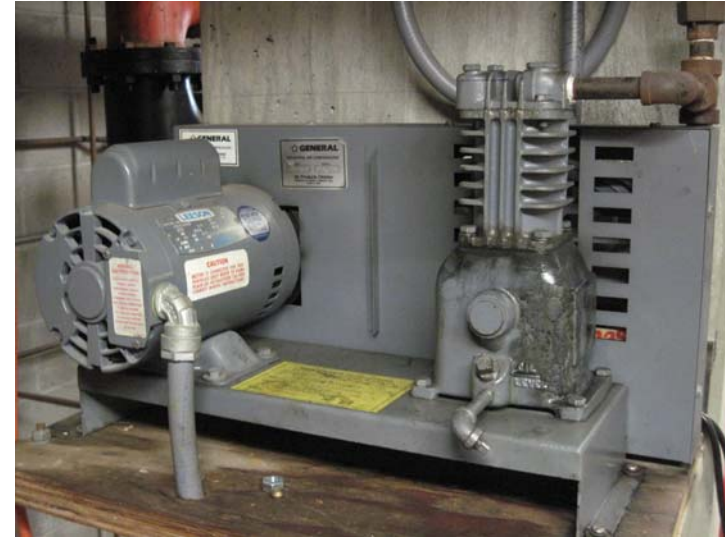
View of the parking garage dry-pipe fire suppression system Leeson 3/4-horsepower compressor.
