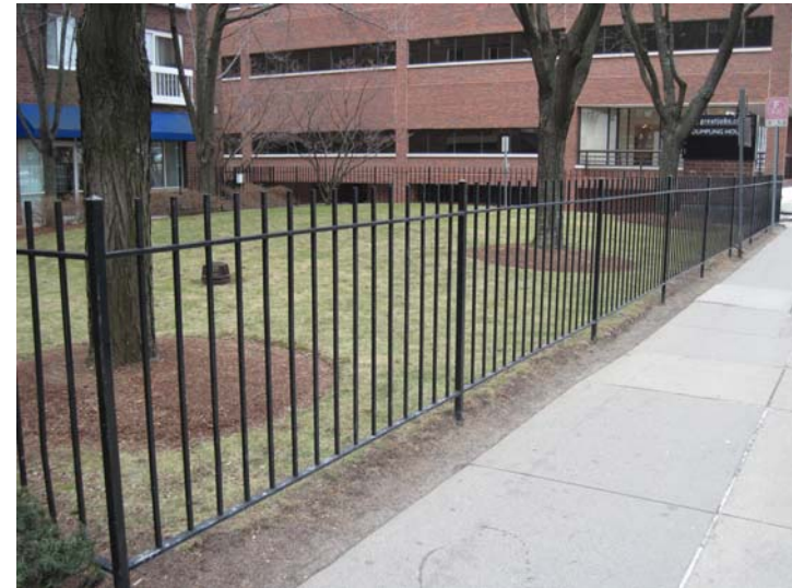
The painted metal fence bordering the front park exhibits overall age and weather-related paint failure; in need of sanding priming, and painting.
