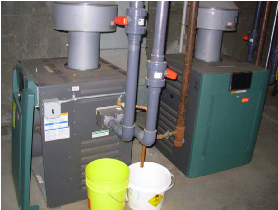
5. RayPak heating boilers serving the pool and spa.
