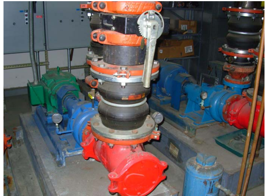
12. Heating-cooling loop circulation pumps.
