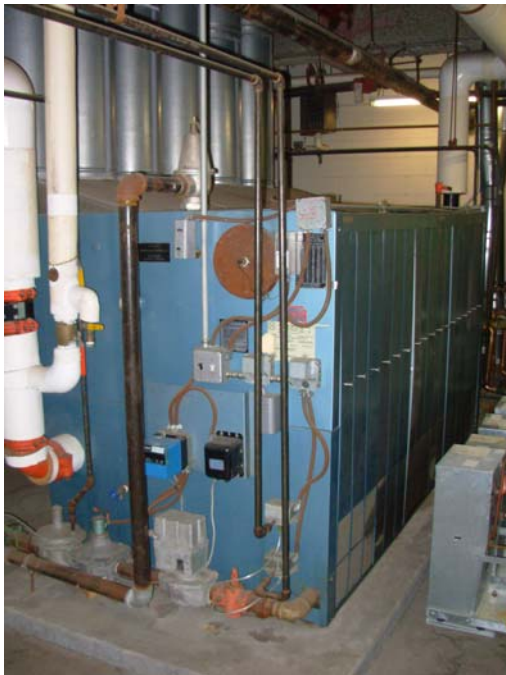
7. H.B. Smith heating boiler plant.
