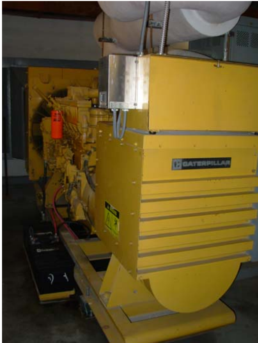
17. View of the Caterpillar emergency generator.
