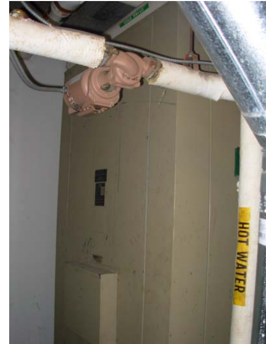
10. Lochivar DHW storage tank, recently re-lined.
