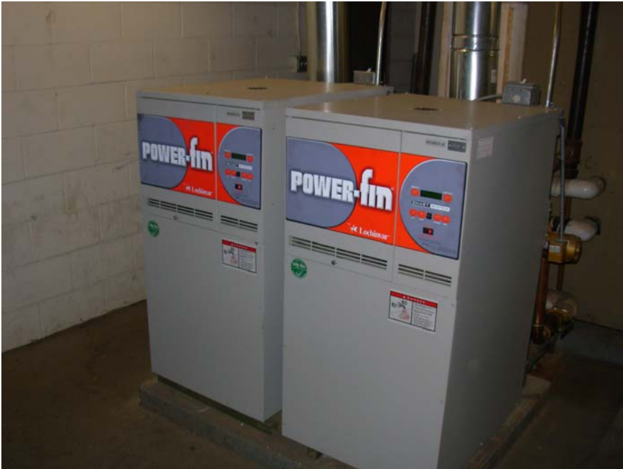
9. Lochivar DHW boilers, recently installed.
