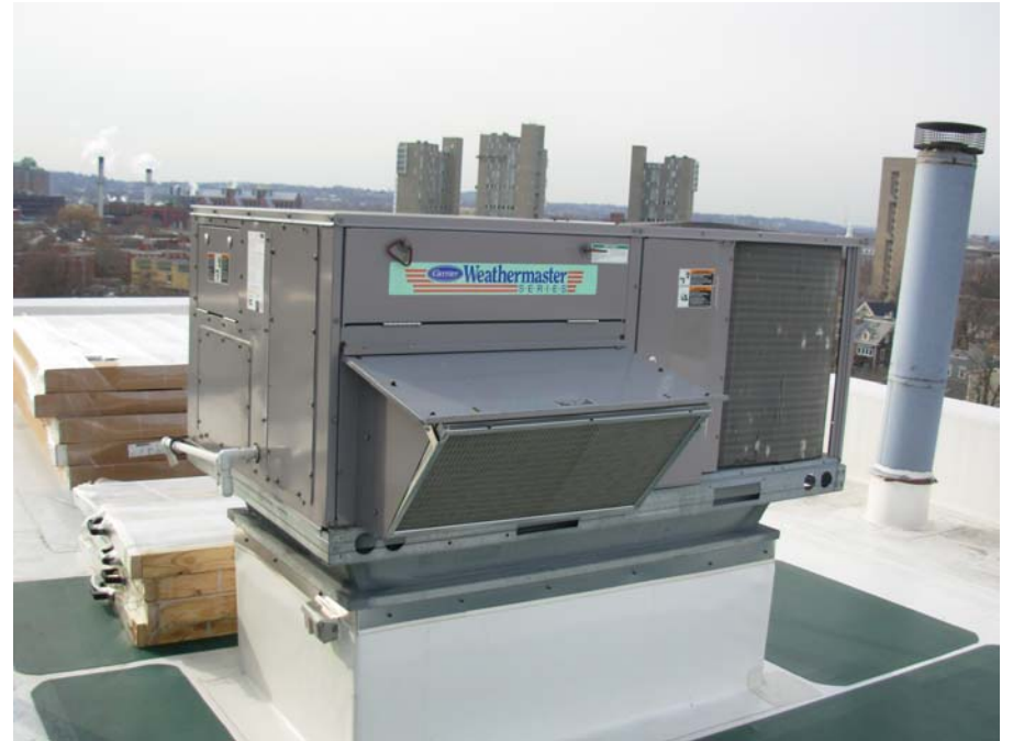
14. Rooftop make-up air packaged units serving common hallways.
