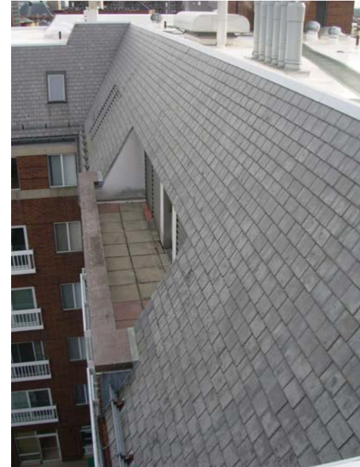
26. Mansard roofing sections.
