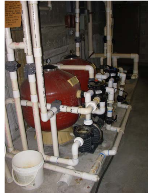
6. Pool and spa filtration and pumping equipment.
