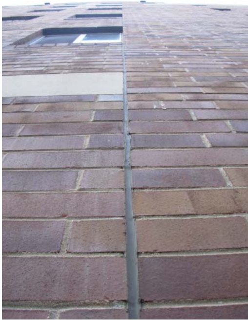
21. Sealant-control joints recently replaced.
