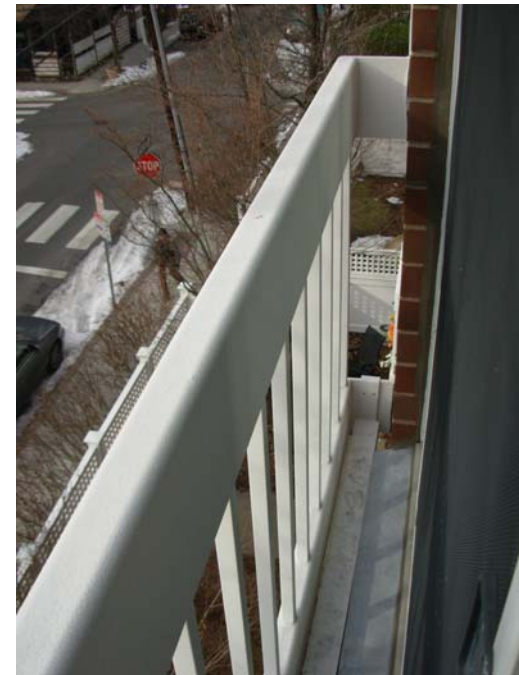
24. Railings recently refinished with Rhinoshield system.
