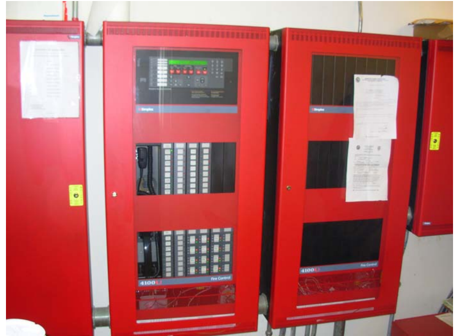
18. Building's main fire detection system monitoring panel.
