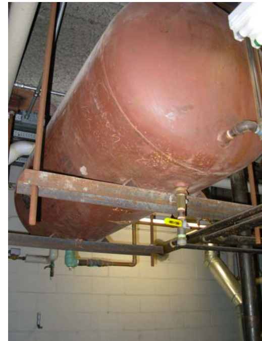
8. Expansion-pressurization tank leaking, to be replaced.
