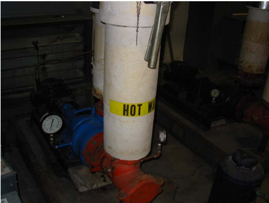
11. Hot water circulation pumps, to be replaced.
