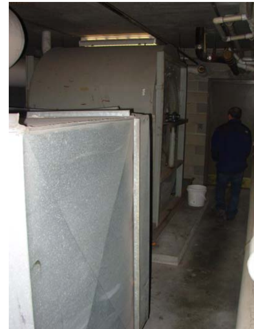
16. Garage intake and exhaust fans.
